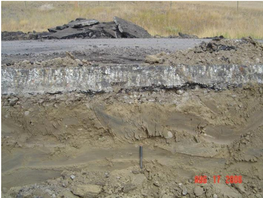
5" Asphalt, + 8" Base (15 yrs old)
