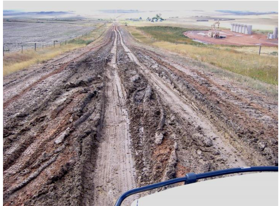
3" Scoria, old gravel base (after 3 months)
