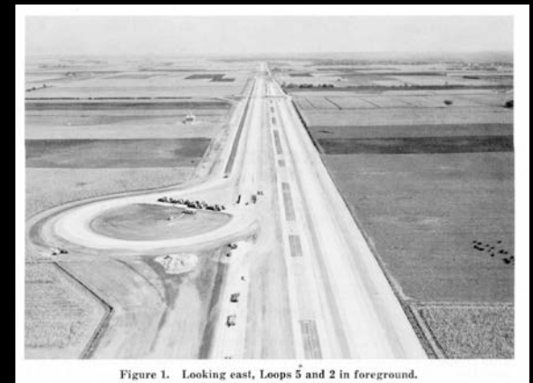
Figure 1. Looking east, Loops 5 and 2 in foreground.
