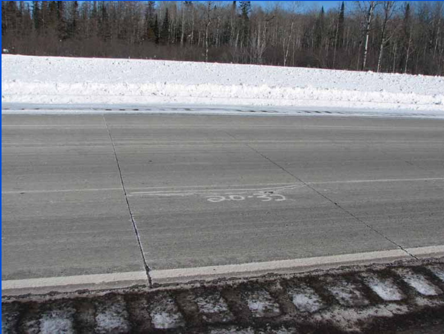
Crack in 6' x 6' panel
