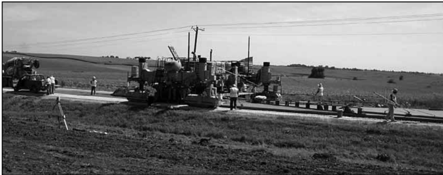
An overlay project (photo: National Concrete Pavement Technology Center)
