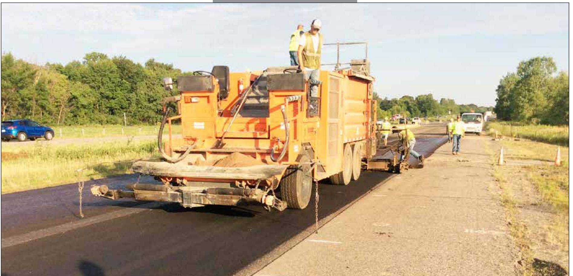
A section of MnDOT's MnROAD test track is microsurfaced as new National Road Research Alliance addresses troublesome paving issues to help DOTs nationwide.
