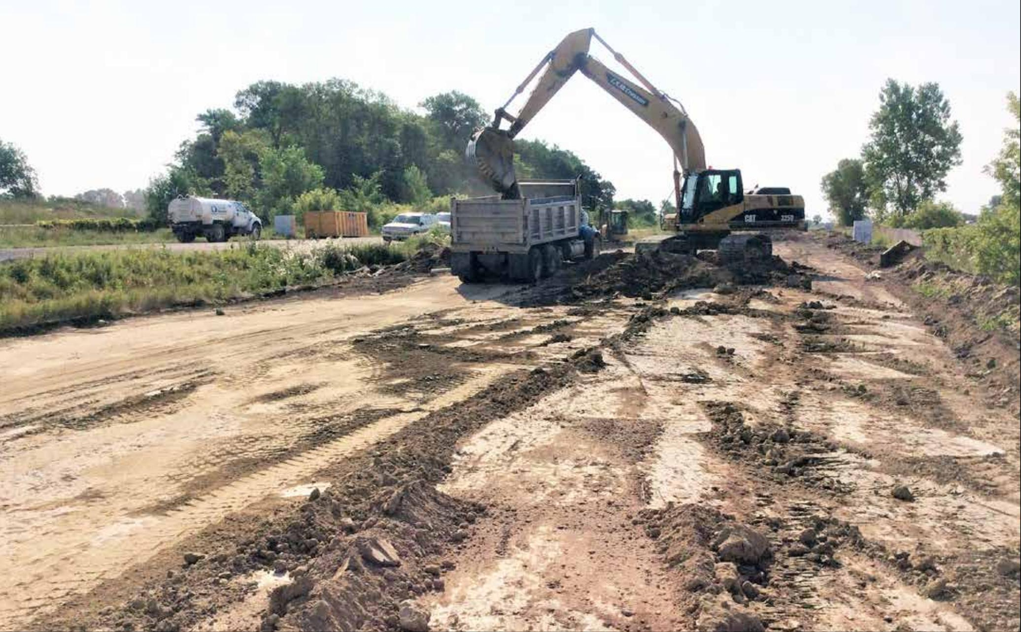
Excavation of new test cell takes place, with clay surface to be subsequently watered to produce mud, then covered by large stone base to see if it will support pavement structure.
