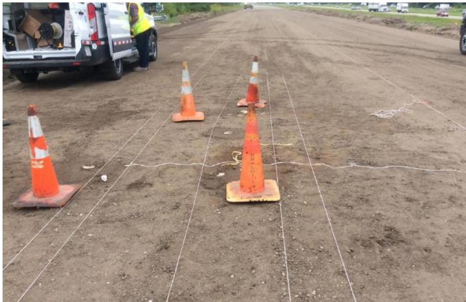
Figure 13: Completed Sub-surface Sensor Installation in Cell 19
