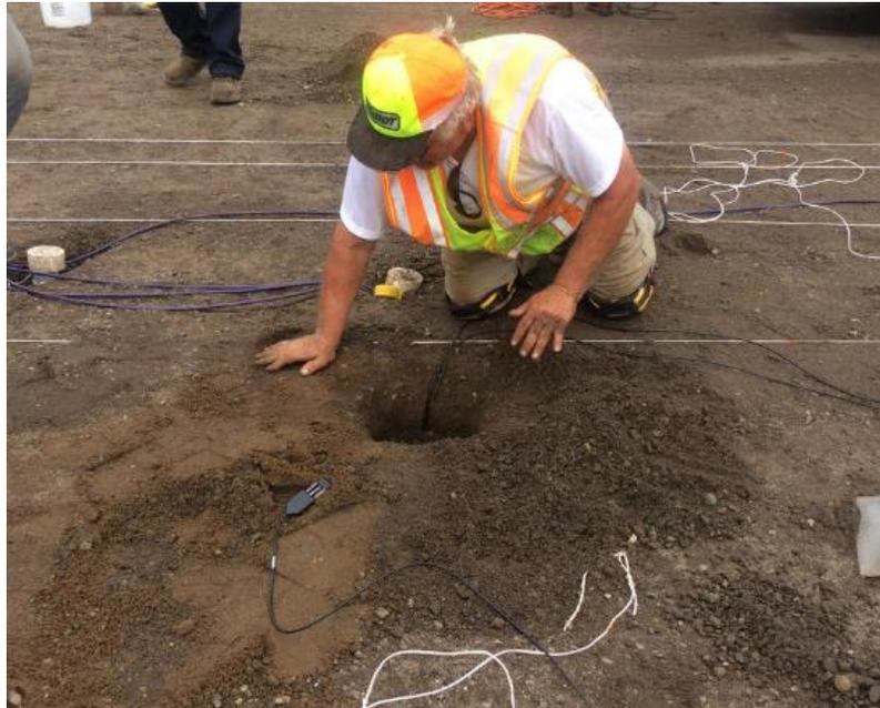
Figure 8: Moisture Sensor Installation
