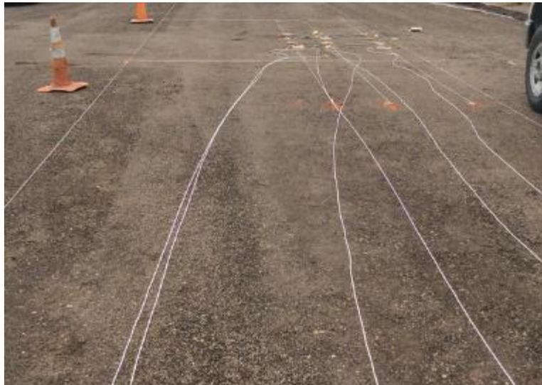
Figure 15: Unrolling of Strain Gauge Wires
