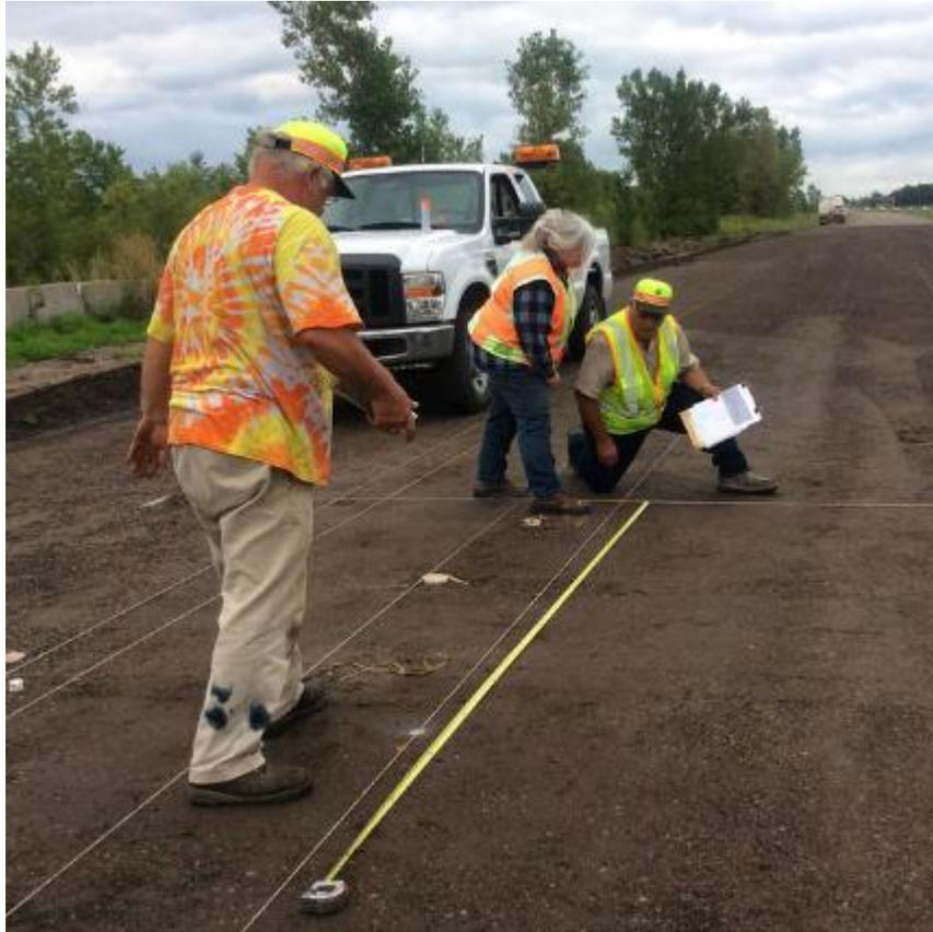
Figure 14: Marking Strain Gauge Locations
