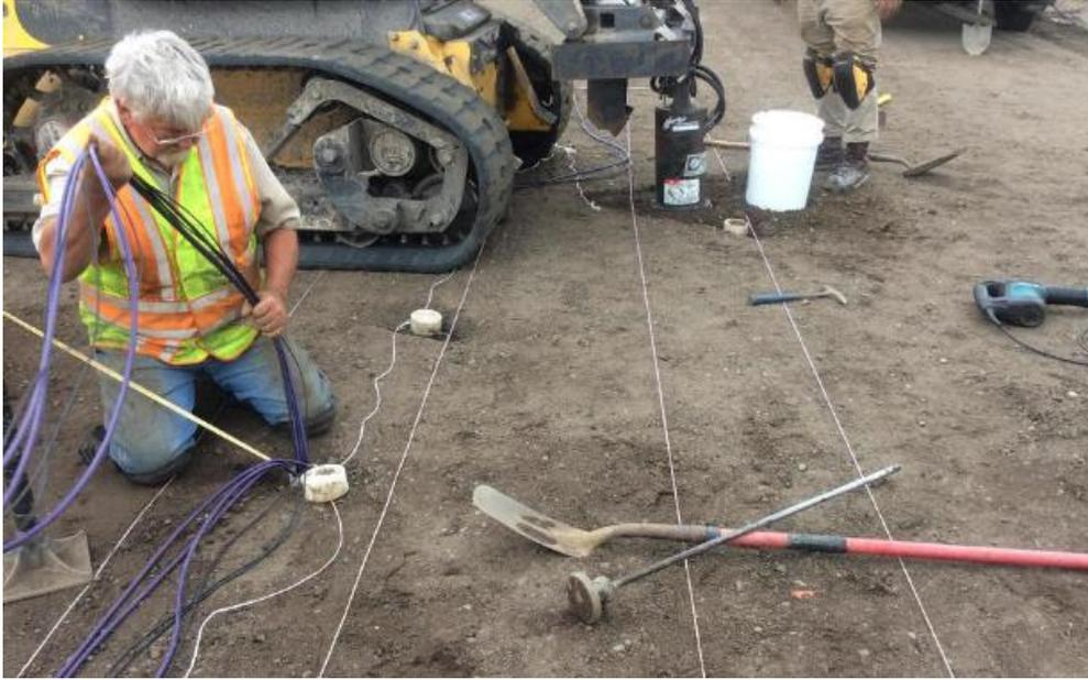
Figure 10: Placing Wires into Conduit
