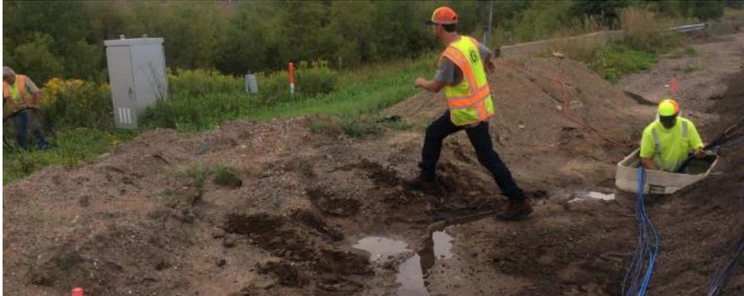
Figure 12: Pulling Wires from Vault to Hand Hole
