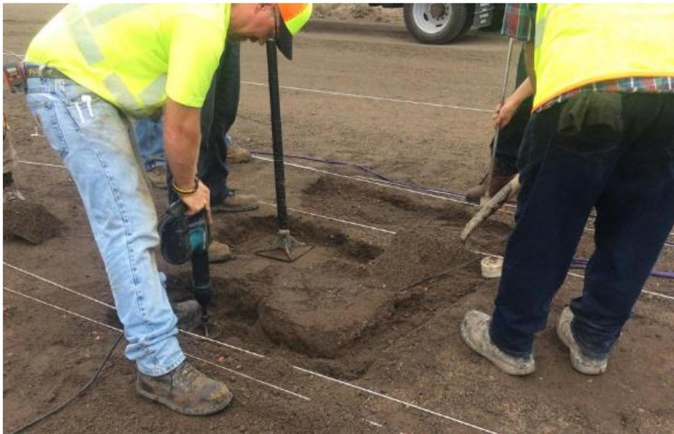
Figure 7: Compaction of Base Above Pressure Gauges
