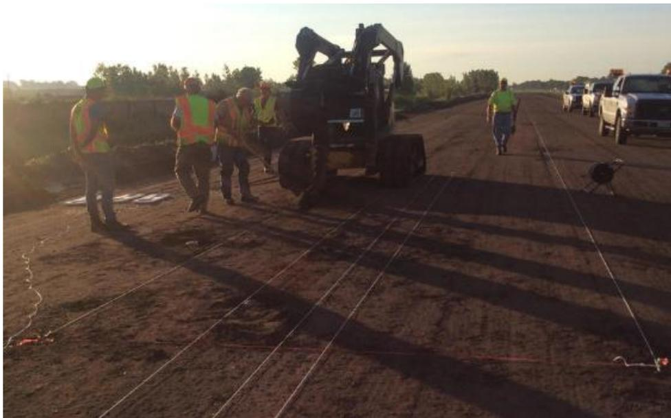
Figure 3: String Line Layout and Trenching for Pressure Gauge Installation
