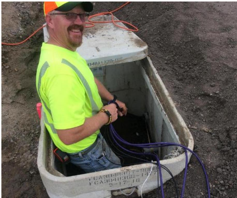
Figure 11: Pulling Wires from Conduit into Vault
