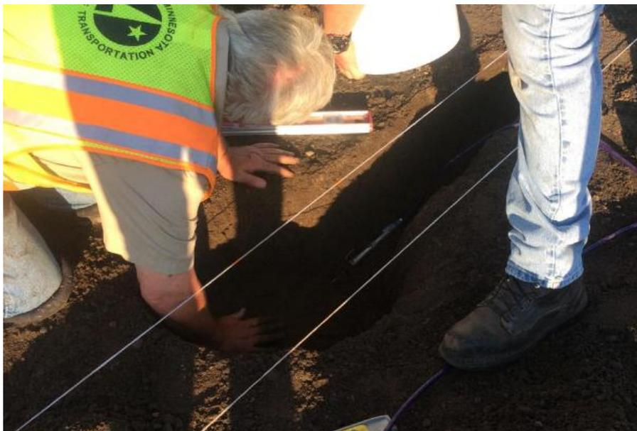
Figure 5: Levelling of Pressure Gauge
