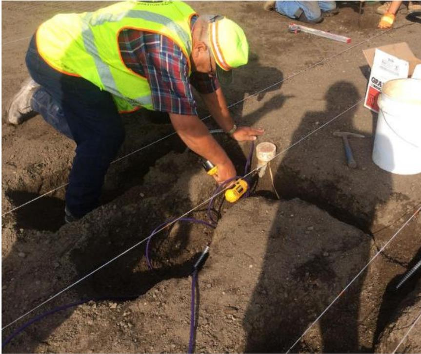
Figure 6: Drilling Hole into Conduit
