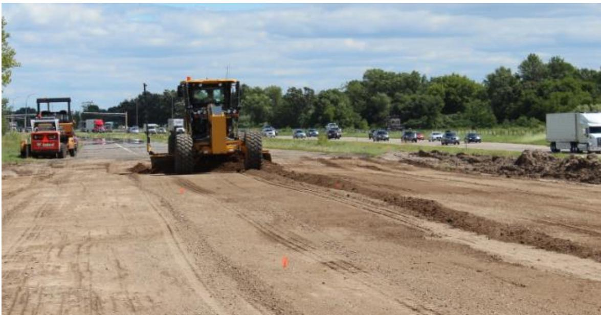
Figure 6: Tolerancing of Subbase
