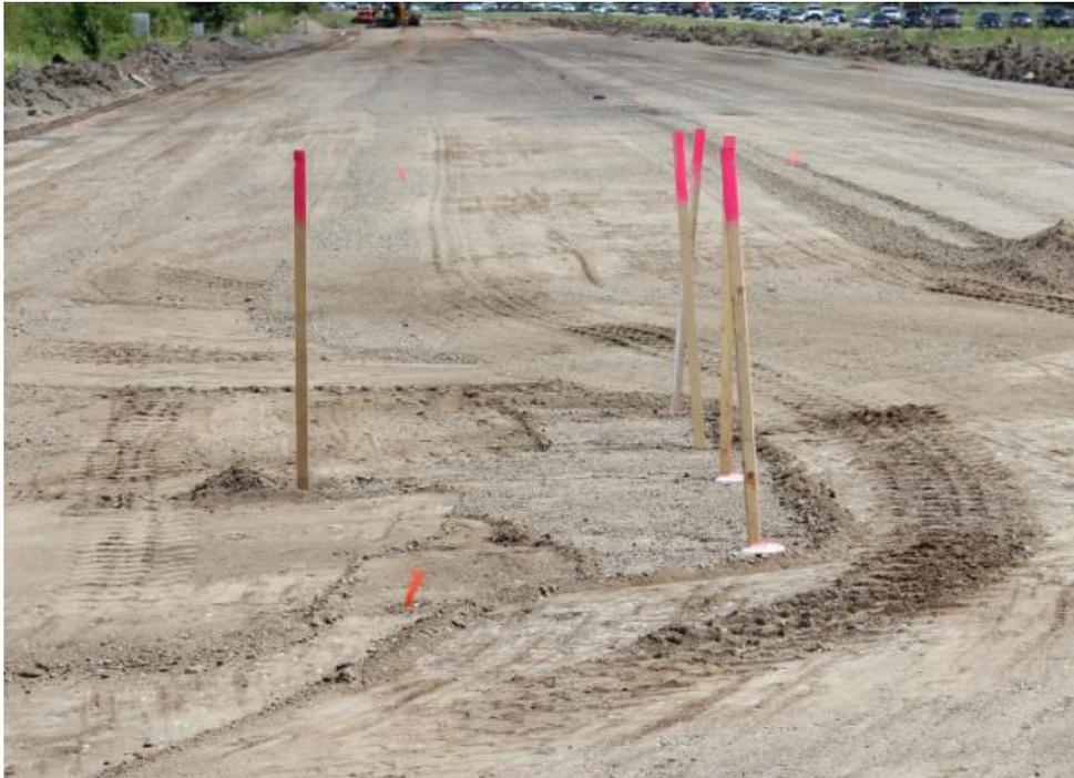
Figure 7: Conduit Marked for Sensor Installation
