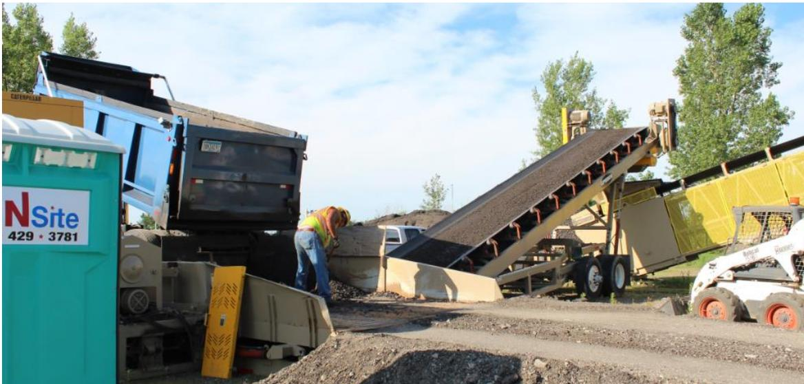
**RAP Material from Haul Truck Transferred into Stacker**
