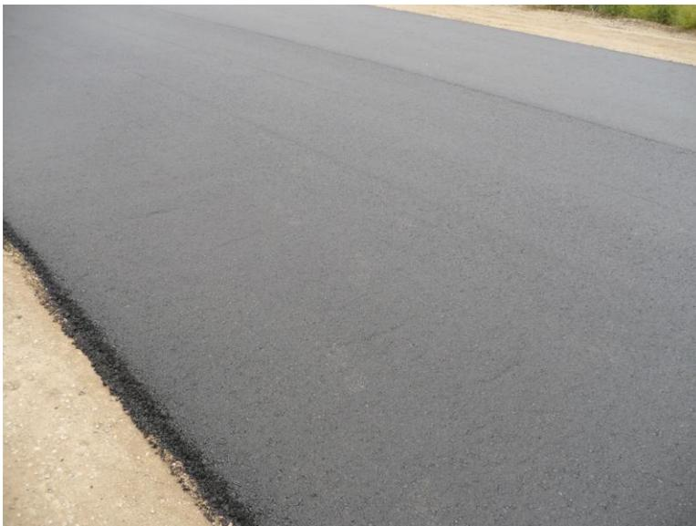
**Figure 22 View of rolled non-wear mixture.**
