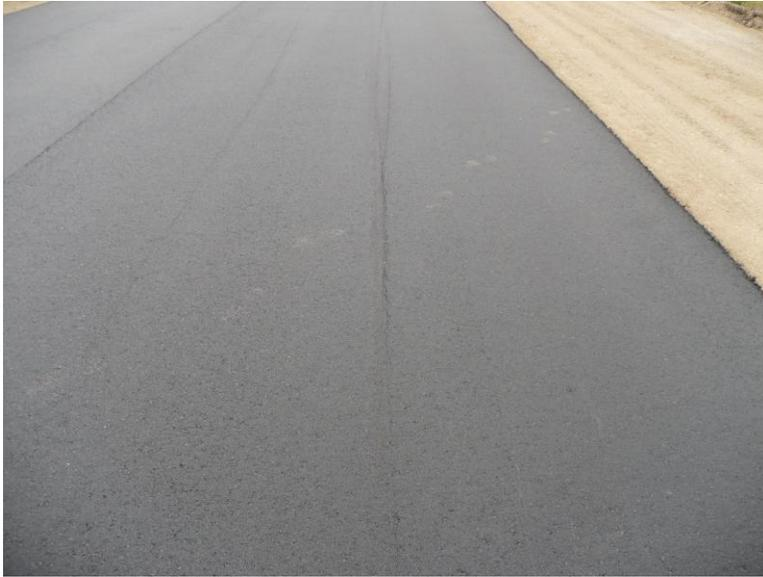
**Figure 21 Longitudinal view of rolling patterns over non-wear mix.**
