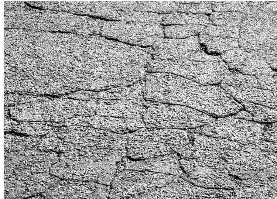
Block Cracking
