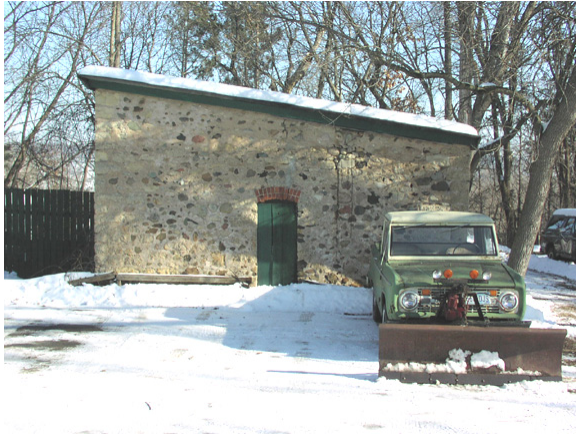
Shoddy Mill-West Elevation
