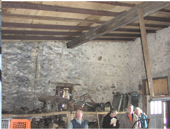
Shoddy Mill-Northwest Interior
