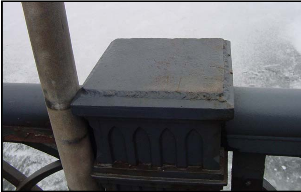
Photo 7: Typical Retrofit of Newel Post Light Anchorage
