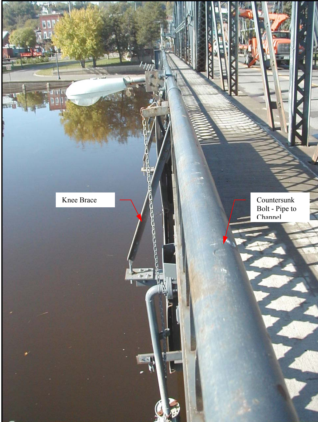
Photo 3: Pedestrian Railing Knee Brace
