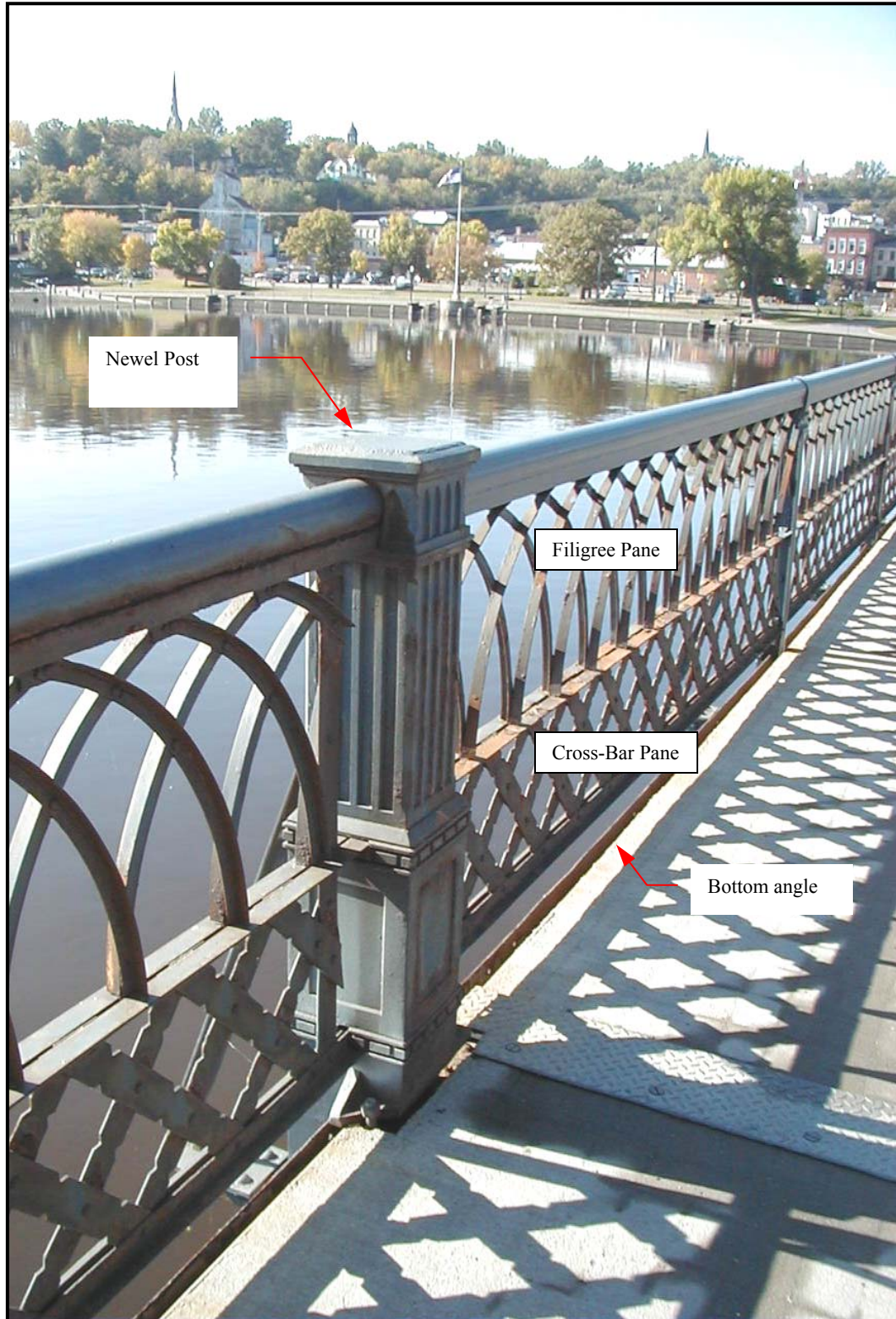
Photo 4: Typical Newel Post, Filigree and Cross-bar Panes
