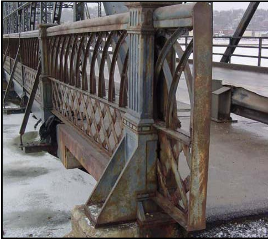
Photo 9: Span 10 Modified Newel Post
