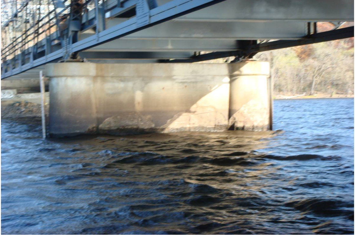
Photograph 7. View of Pier 8, Looking Southeast.
