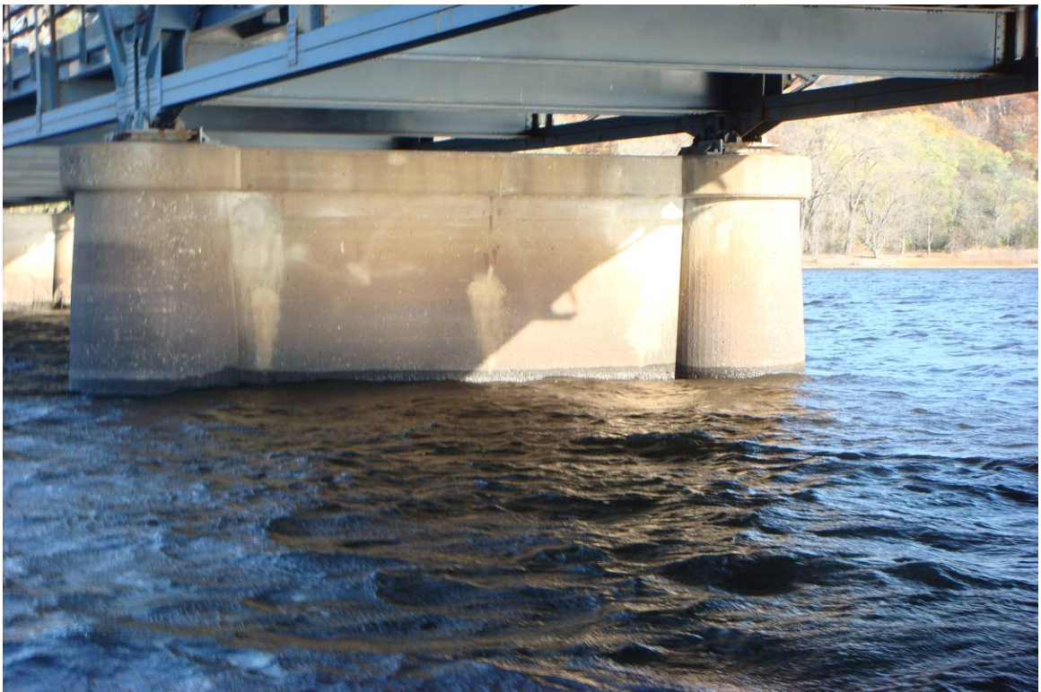
Photograph 6. View of Pier 7, Looking Southeast.
