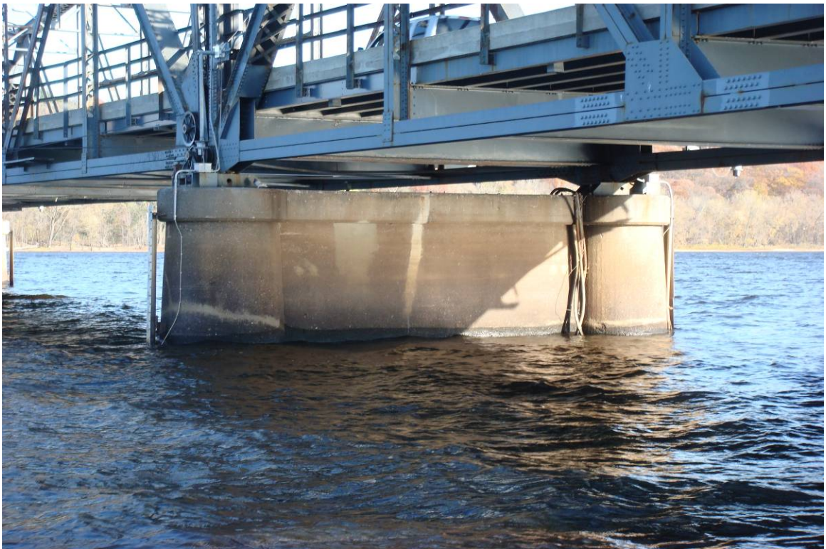
Photograph 2. View of Pier 3, Looking Southeast.
