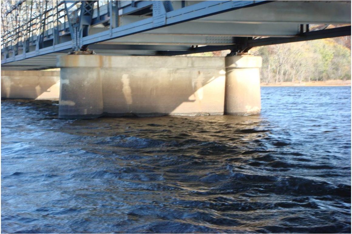
Photograph 5. View of Pier 6, Looking Southeast.
