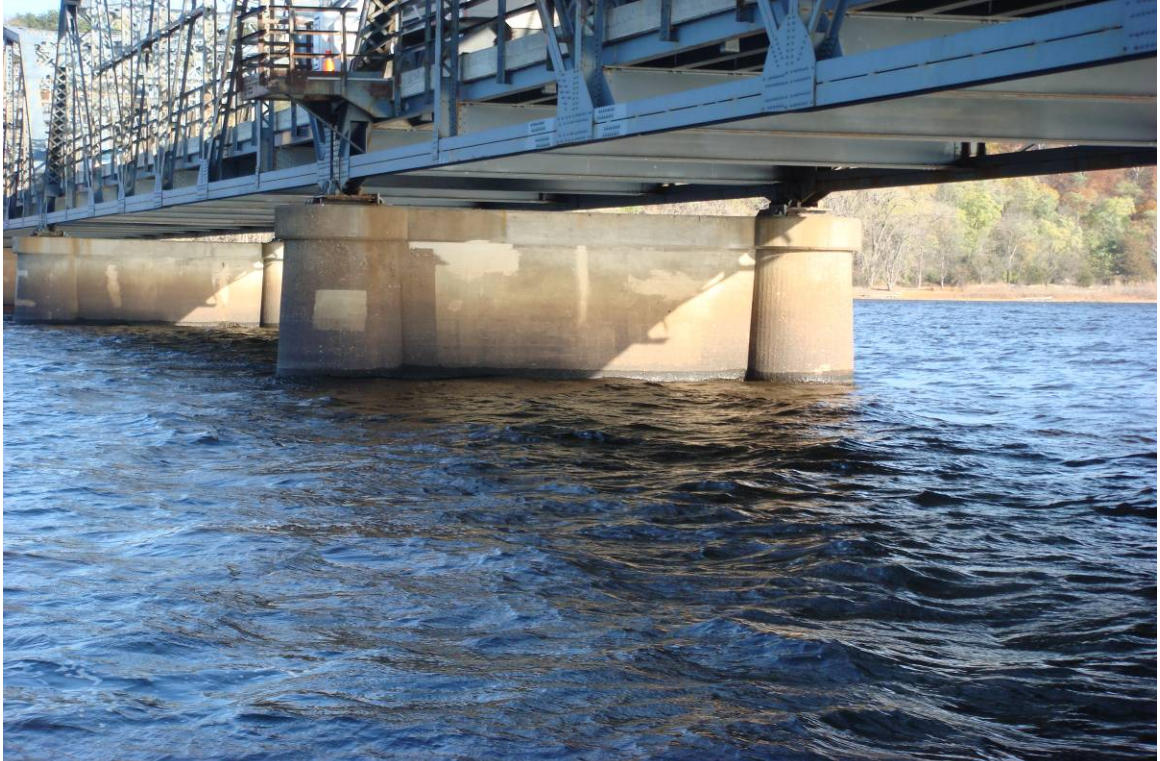
Photograph 4. View of Pier 5, Looking Southeast.
