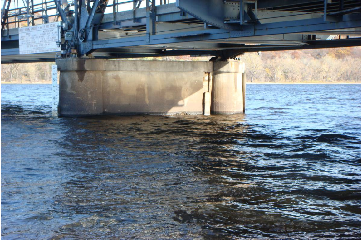
Photograph 3. View of Pier 4, Looking Southeast.
