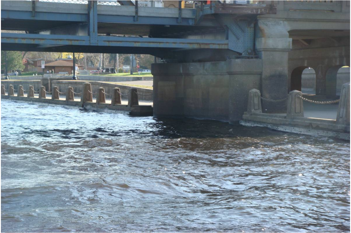
Photograph 1. View of Pier 2, Looking Southwest.
