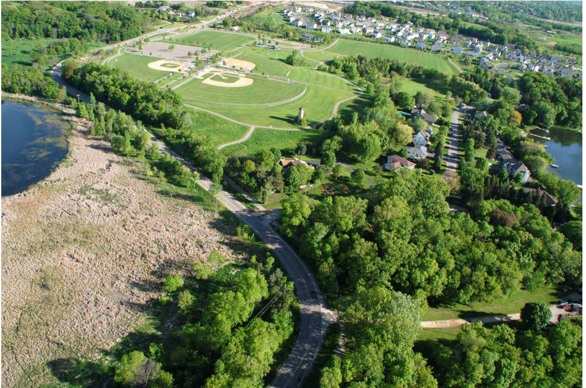
Hwy 101 at Kiowa Trail looking north
