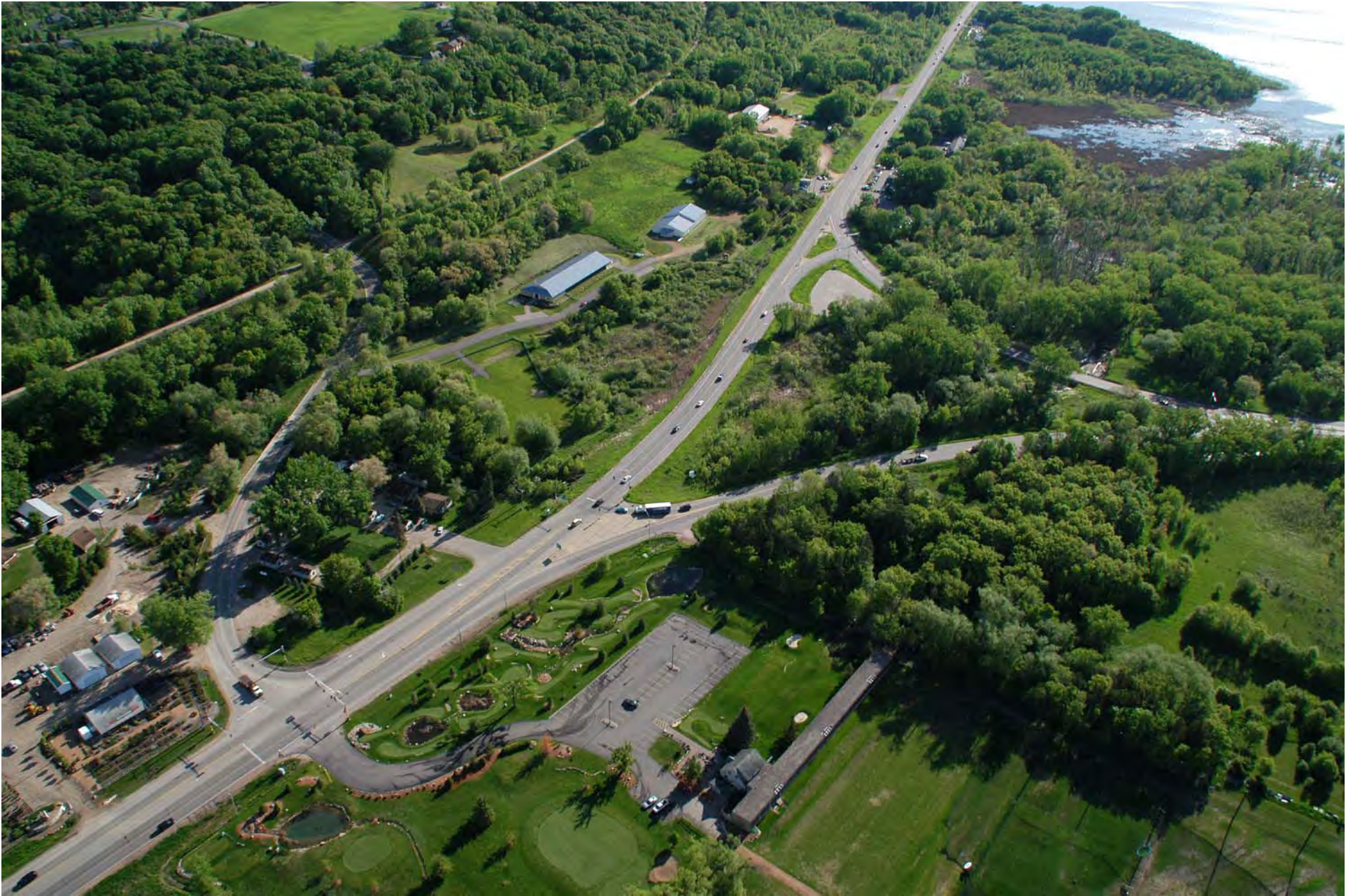
TH 101 Jct. with TH 212 – Looking East
