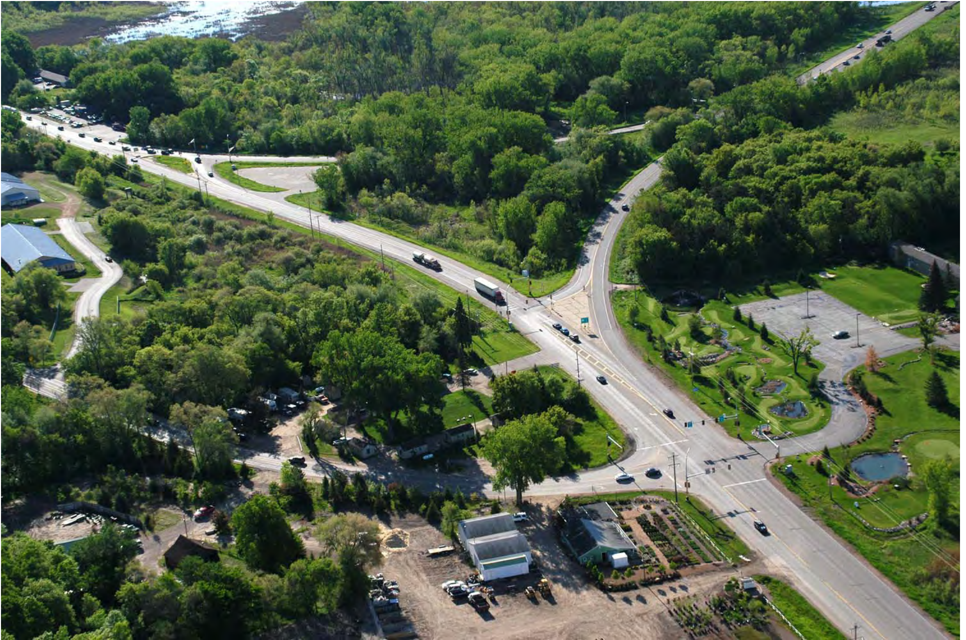
TH 101 Jct. with TH 212 – Looking SE
