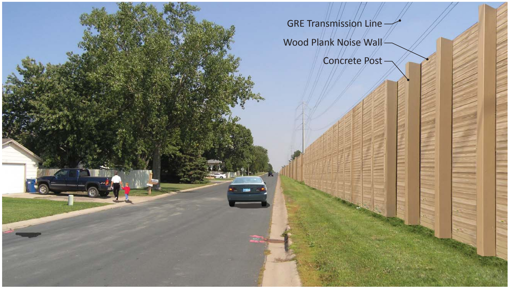
View of Proposed Noise Wall on 97th Avenue Looking East from Hemlock Lane
