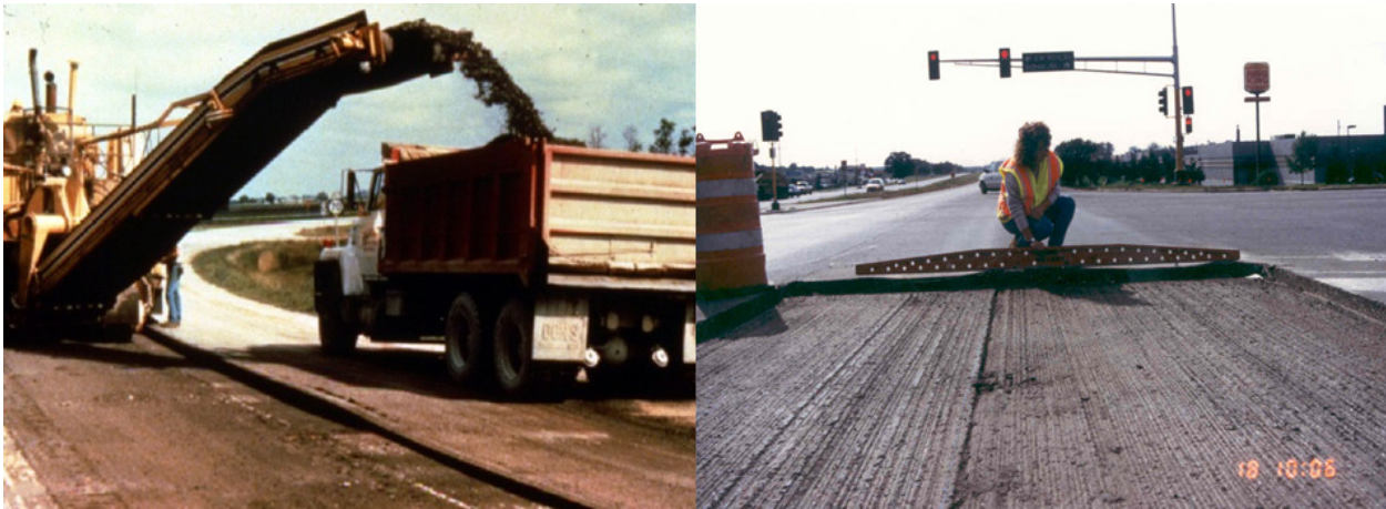
Figure 7. Asphalt milling operation and the HMA surface after milling.
