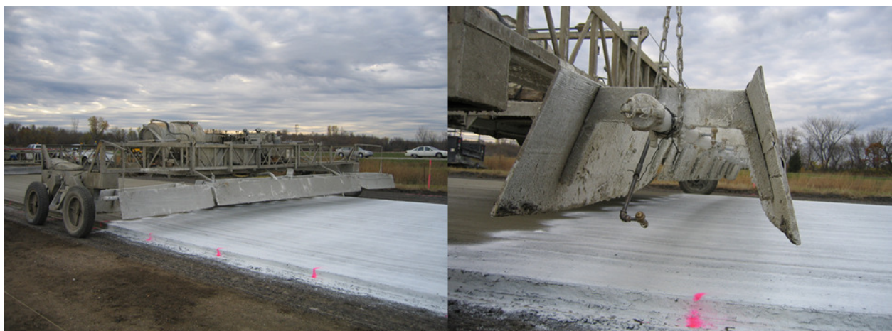
Figure 9. Application of a curing compound.
