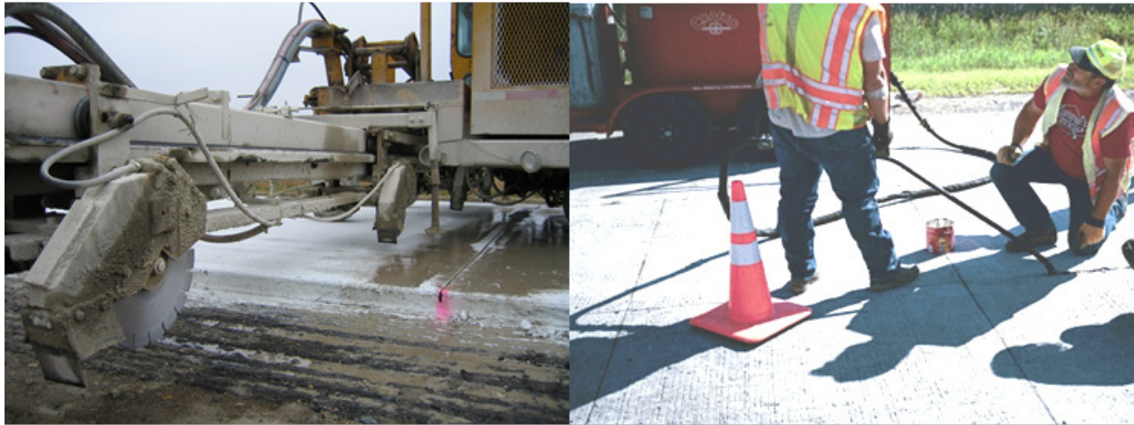
Figure 10. Sawing and sealing joints.
