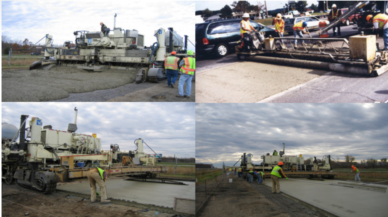
Figure 8. Placing and finishing the BCOA.
