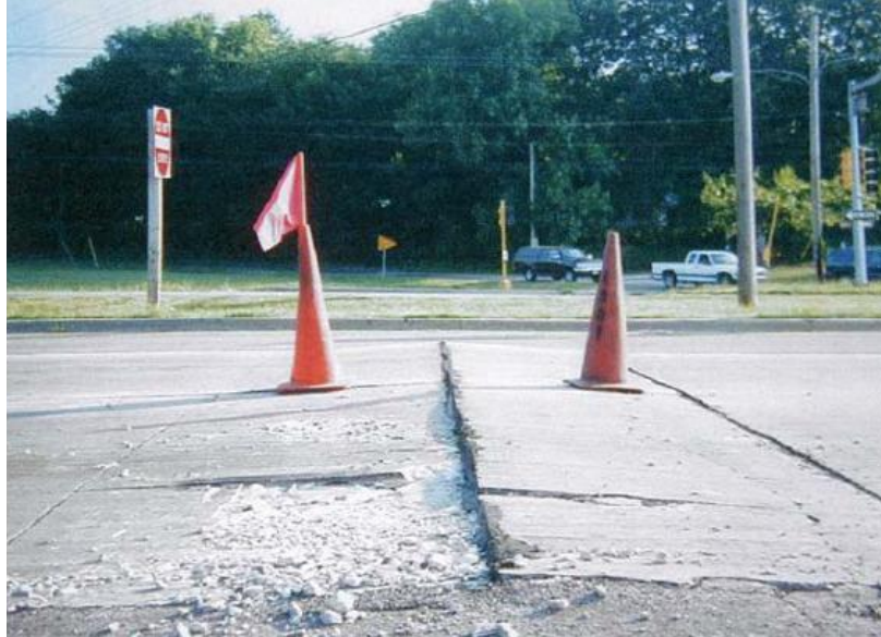
Figure 46: Blow up of the UTW slabs (Winkelman, 2005).
