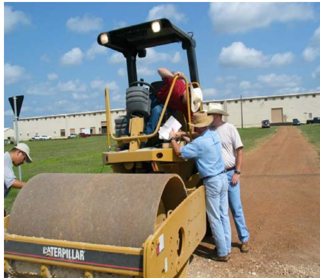
Figure 14. Preliminary Field Testing of Instrumented Roller.
