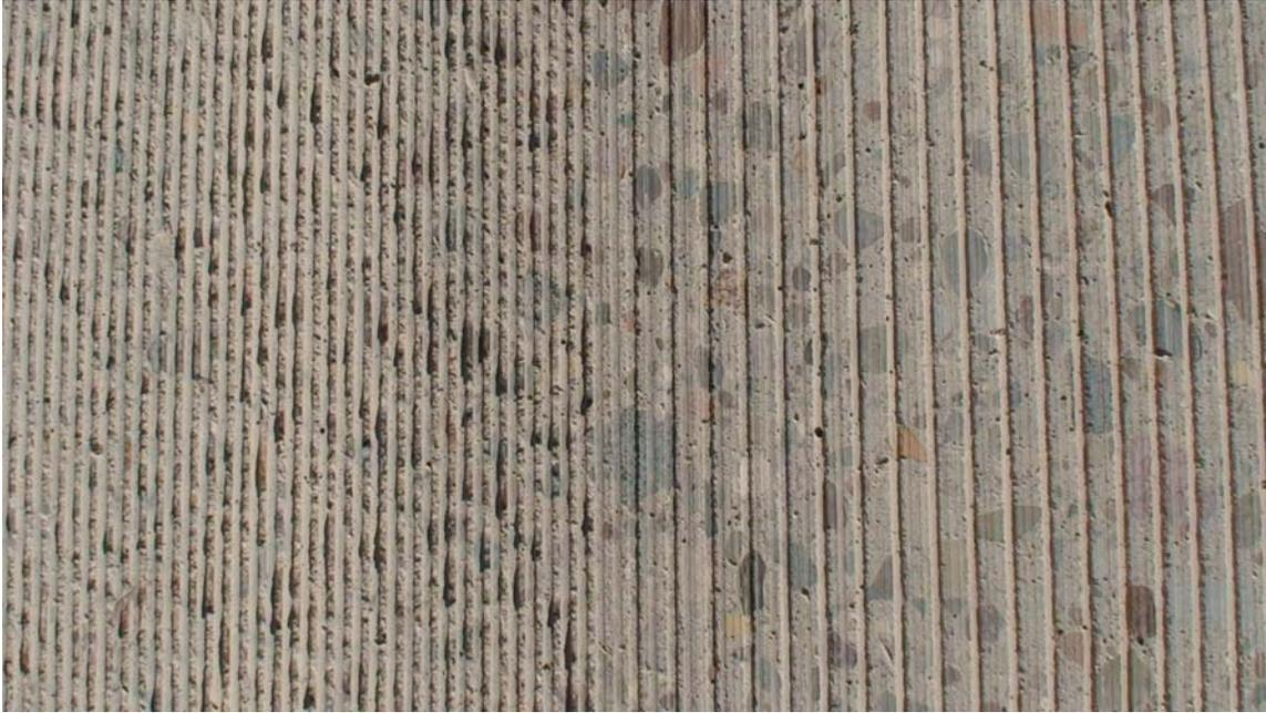
Fig 4.3 Conventional Grind and Innovative Grind
