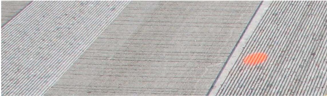
**Fig 3.2.2 Close-up View of the Quiet Configurations TS1 and TS 2 With Original Transverse tine texturing sandwiched between.**
