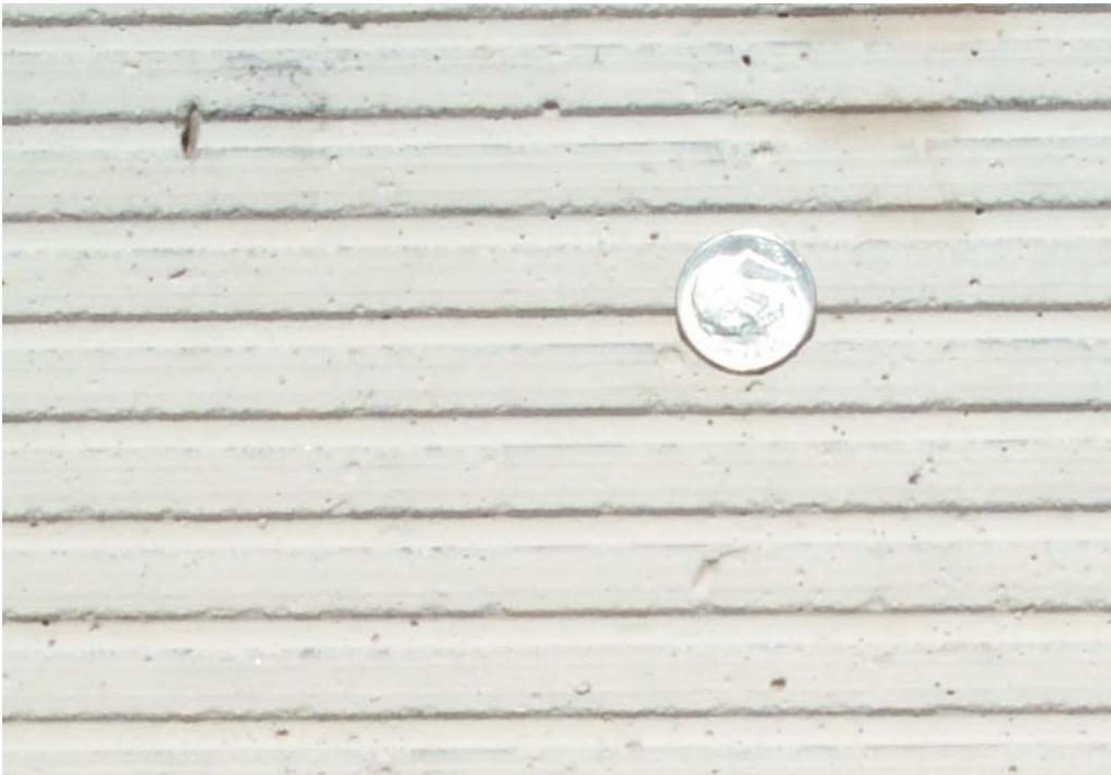
**Fig 3.2.4 Close-up View Of TS1 Innovative Grind in one pass Cell 37 MnROAD**
