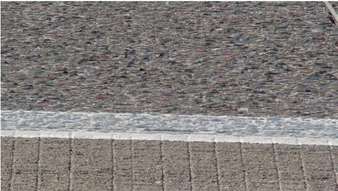
Fig 4.4 Conventional Grind Cell 8 And Previous Texturing (Transverse Tine)
