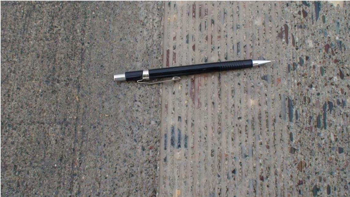
Fig 4.2 Conventional Grind Configuration (0.125X 0.125x.0.120)
