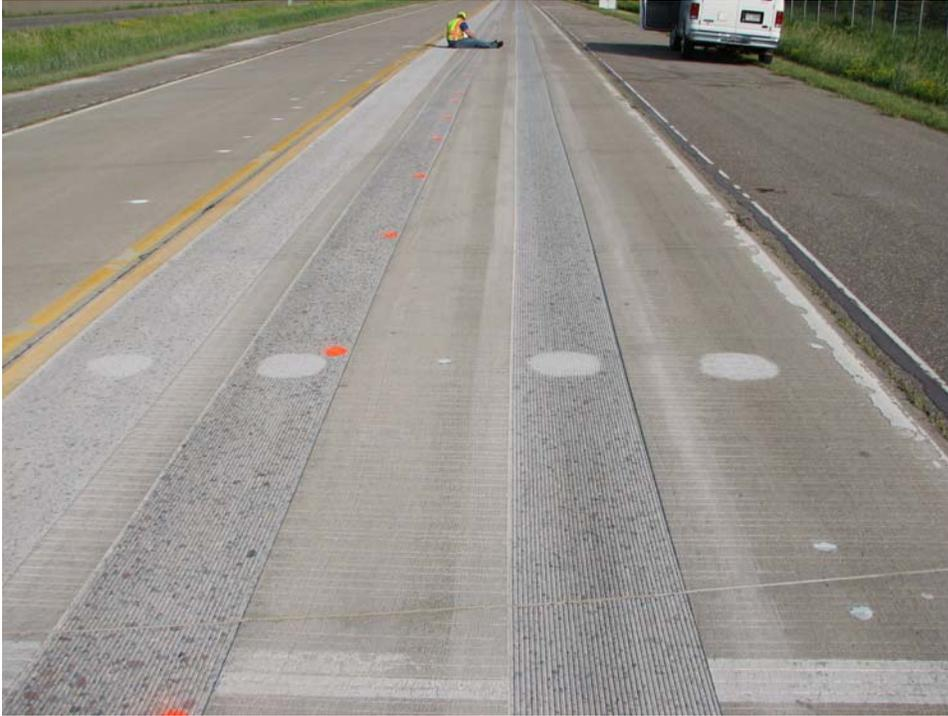
**Fig 3.2.3 A Panoramic View of the texture Strips Looking West on Cell 37 MnROAD**
