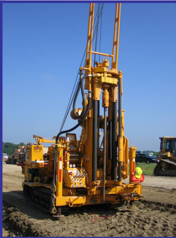
Mn DOT Drill Rig
