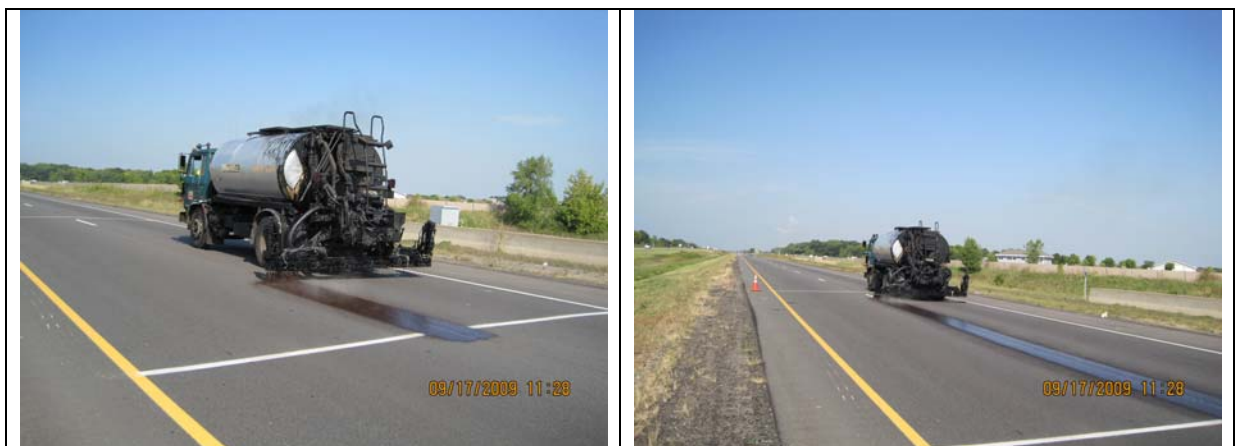
Figure 1. T.H. 94, September, 2009 – 0.10 gal/SY CSS-1h Fog Seal
