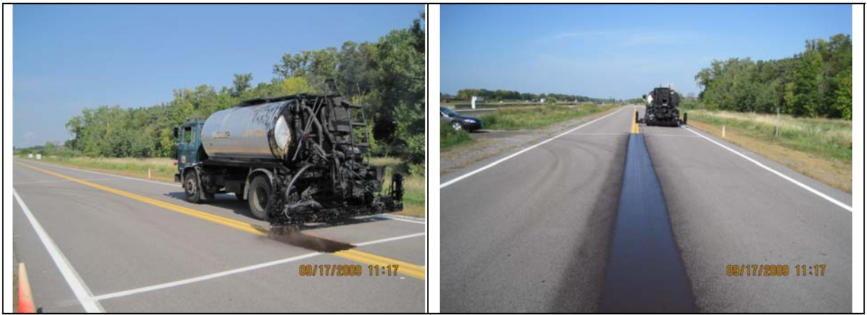
Figure 6. MnROAD CSS-1h Fog Seal applied at 0.10 gal.SY, September, 2009
