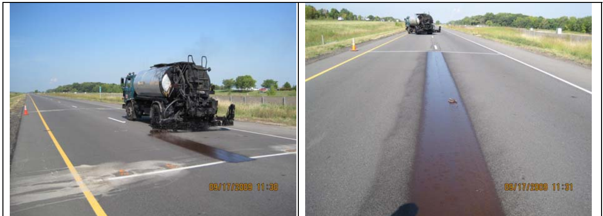
Figure 2. T.H. 94, September, 2009 – 0.15 & 0.20 gal/SY CSS-1h Fog Seal
