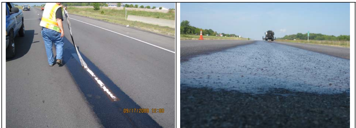
Figure 3. T.H. 94, CSS-1h Fog Seal after 25+ minutes, September, 2009
