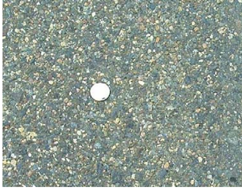
Otta Seal constructed 2001, Cass County CR171.
