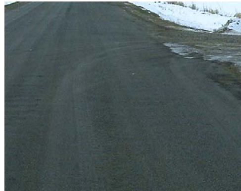
Otta Seal constructed 2001, Cass County CR25 – Dairy Farm.
