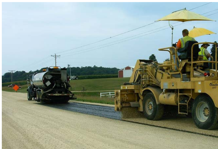
Otta Seal Const. 2007, Olmsted County CR58
