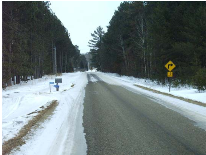
Otta Seal constructed 2003, Cass County CR168.
