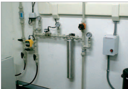
The liquid dispensing and blending unit uses a series of pumps equipped with flow meters.
