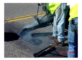
**Background:** There are many miles of bituminous roadways that are not meeting customer criteria do mainly to thermal cracks creating a rough ride. This is unacceptable by consumers and repairs need to be completed.
