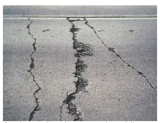
> ½ inch). Measurement of distress is made for observed cracks over a selected distance. Detailed guidance on measurement techniques is contained in the MnDOT and FHWA Pavement Preservation Manuals referenced earlier.
