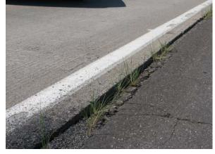
example of an unsafe drop-off condition is shown in <u>Figure 29</u>. Shoulders are not designed to carry heavy traffic and improper use can cause extensive damage. Maintenance of shoulders and approaches is influenced by their design, condition and
