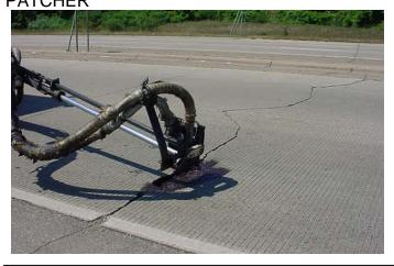
Patching may also be injection using а spray done technique ("blow patching") where air pressure is used to apply a mix of fine aggregate and asphalt emulsion into potholes or large cracks. Still another effective patching technique involves the use of mastics which are a proprietary blend of asphalt sealants and aggregate. Specifications for patching materials and procedures are covered in MnDOT specifications and special provisions available from MnDOT Materials Engineering
