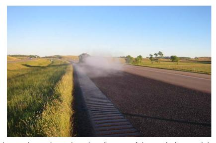
as pavement friction (skid resistance) may be reduced until some of the asphalt material is worn off. Information on application techniques and material rates can be found in the Minnesota Seal Coat Handbook 2006, the MnDOT Best Practices Handbook for Asphalt Pavement Maintenance, and the MnDOT Distress Identification Manual. Fog sealing of a road shoulder is illustrated in Figure 3.
