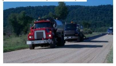
Chip seals or seal coats are applications of asphalt followed immediately with an aggregate cover layer. Applications with two layers are referred to as double chip seals. Seal coats are primarily used to protect the pavement from the deteriorating effects of sun (asphalt hardening and oxidation or "chalking") and
