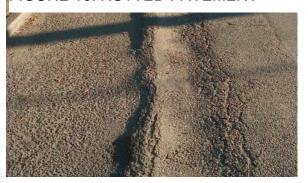
Figure 11. Microsurfacing with a slurry mix or use of mastic material could be considered an alternative to tight blading (see Section 3-4.04.01.05 above for information on microsurfacing).
