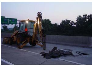
FIGURE 17: BLOW-UP REPAIR
