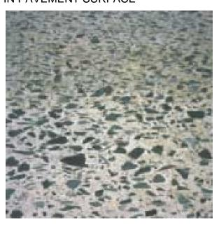
FIGURE 26: SCALING OF CONCRETE SURFACE
