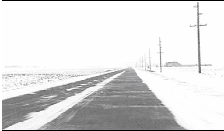
End of Clean-up Operation Figure 2-3.02B
