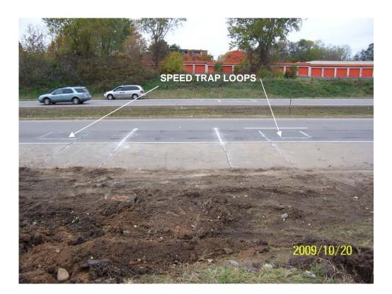
Figure 2 Typical WIM Site Speed Trap (Source: Mn/DOT files) Please see the corresponding *Minnesota Statewide Regional ITS Architecture and Systems Engineering Checklist (Checklist)* for the project locations.
