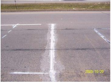
PIEZO QUARTZ SENSOR INSTALLATION
