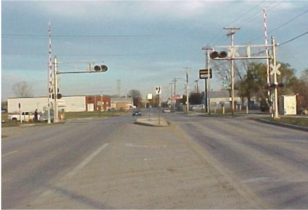
Figure 5 Standard Railroad Gates – With Median (Source: Public Utilities Commission of Ohio Grade Crossing Inventory, http://www.ohiorail.ohio.gov/crossings.php )
