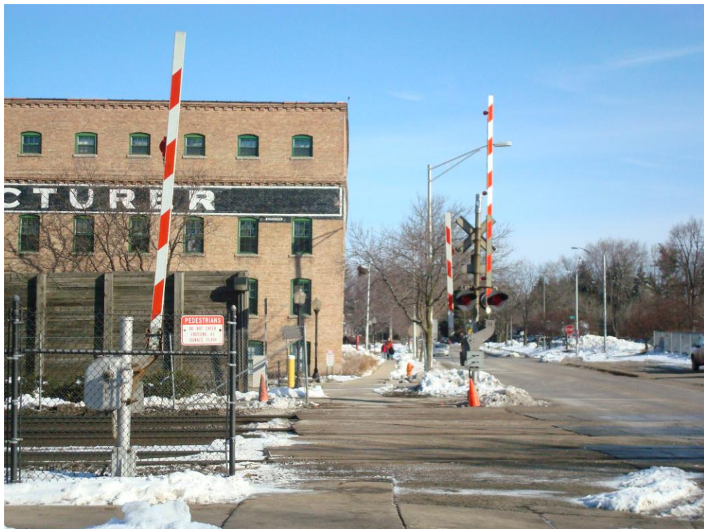
Figure 4 Standard Railroad Gates with Pedestrian Gates
