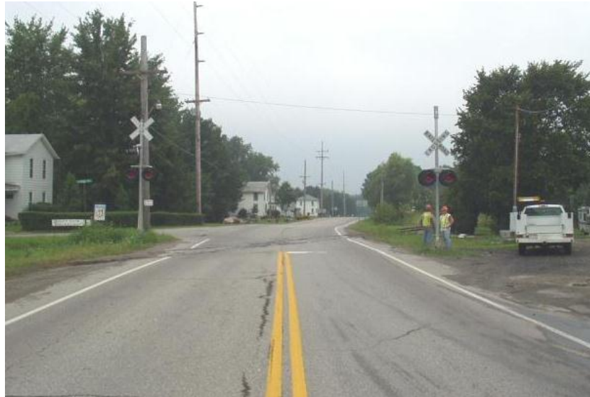
Figure 1 Typical Flashing-Light Signals
