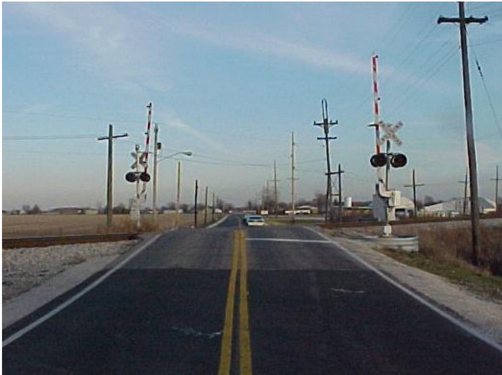
Figure 3 Standard Railroad Gates
