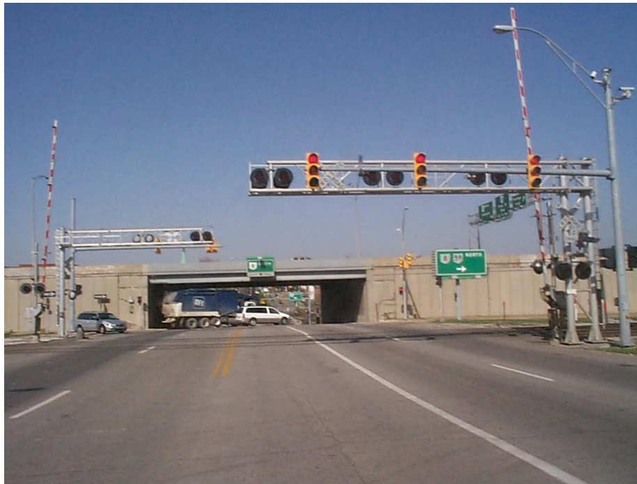
Figure 7 Grade Crossing with Traffic Signal Preemption (Source: Public Utilities Commission of Ohio Grade Crossing Inventory, http://www.ohiorail.ohio.gov/crossings.php )
