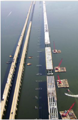
I-10 Bridges, Pensacola, Florida (Flatiron)
