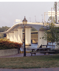
Sagadahoc Bridge, Maine (Flatiron-FIGG)
