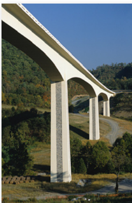
Smart Road Bridge near Blacksburg, Virginia (FIGG)
