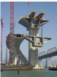
San Francisco-Oakland Bay Bridge, San Francisco, California (Flatiron-Manson)
