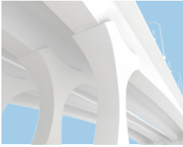
Multiple box girders provide redundancy
