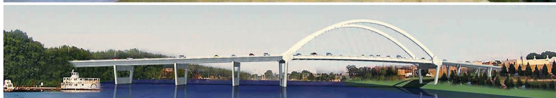
PHOTO: Cretex Concrete Products; RENDERING: Minnesota Department of Transportation
