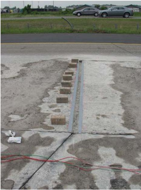
**PIEZO QUARTZ SENSOR INSTALLATION**
