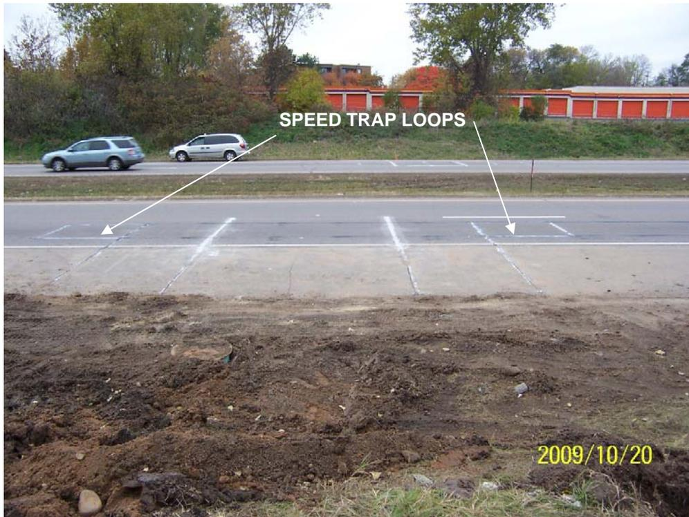
**Figure 2 Typical WIM Site Speed Trap**
