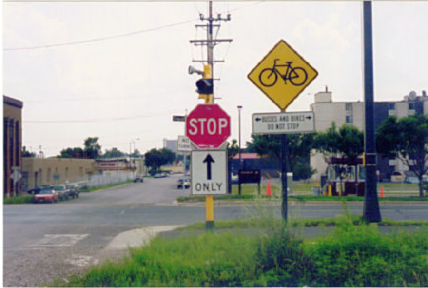
Figure 4. View of the STOP sign and red warning lights at 25th Ave. SE and Transitway.
