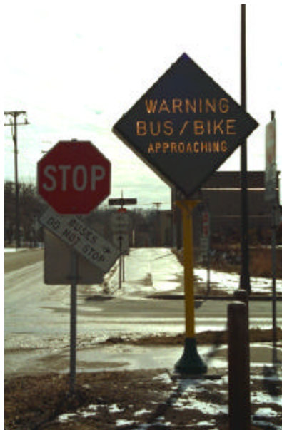
Figure 7. View of the STOP sign and fiber optic warning sign at Malcolm and Transitway.
