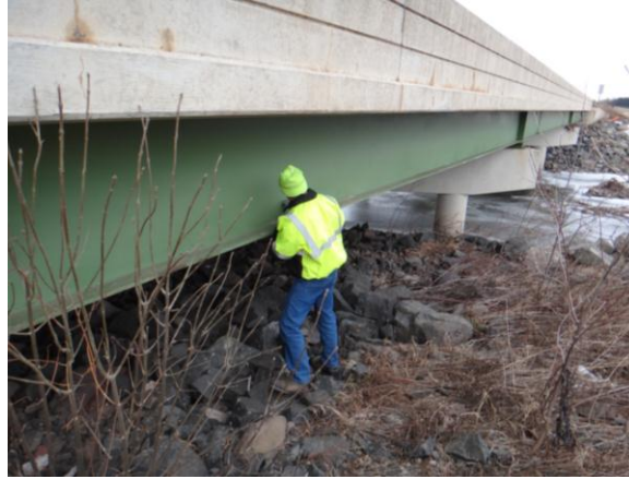
Figure 3.1.11: Bridge #9339 sampling location with waterway
