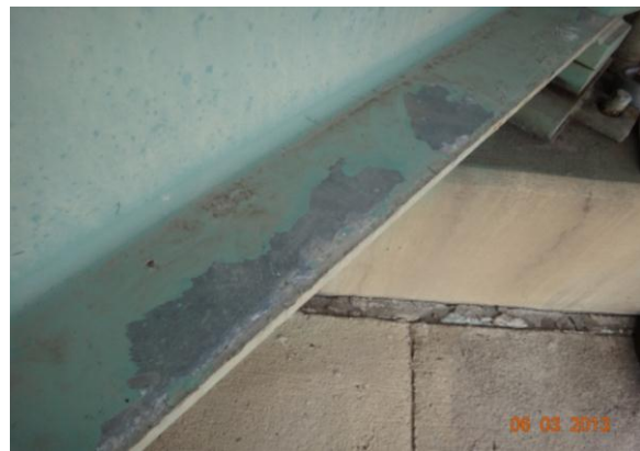
Figure 3.1.6: Bridge #9188 sampling location
