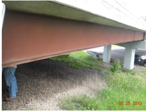
Figure 3.4.48: Bridge #19889 sampling location with roadway
