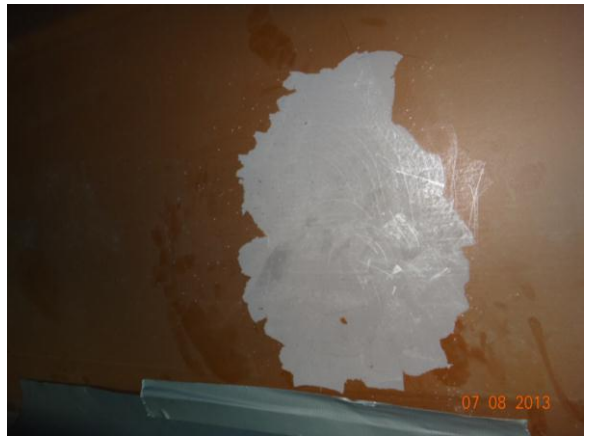
Figure 3.4.35: Bridge #9352 sampling location
