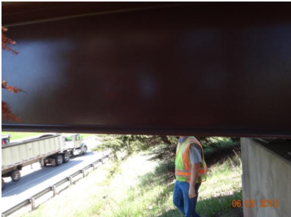
Figure 3.1.9: Bridge #69811 with roadway
