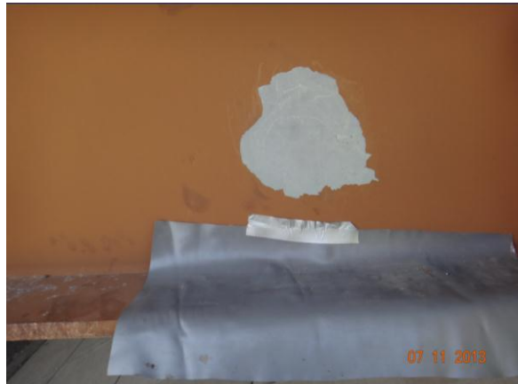
Figure 3.4.12: Bridge #27033 sampling location
