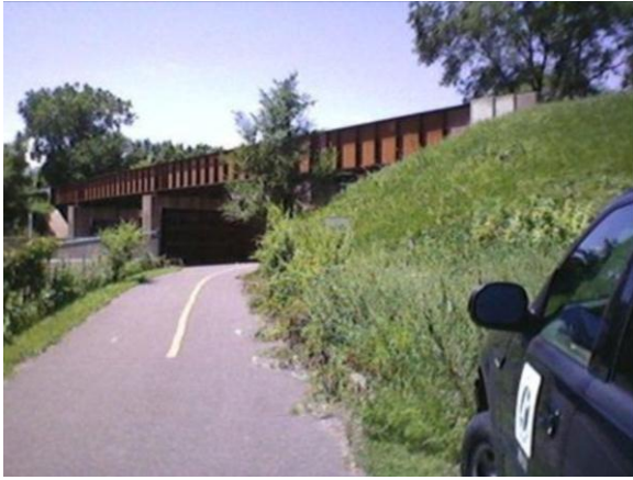
Figure 3.4.36: Bridge #9390 with roadway
