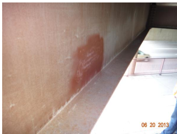
Figure 3.4.21: Bridge #27924 sampling location with roadway
