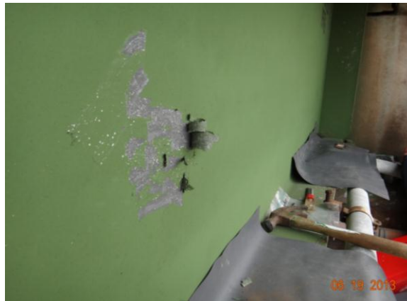
Figure 3.4.59: Bridge #27517 sampling location
