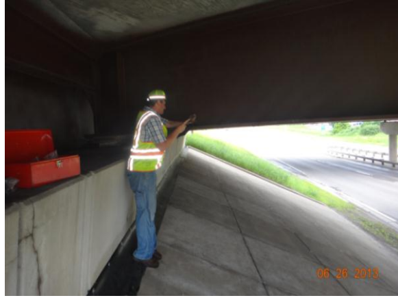
Figure 3.4.56: Bridge #19038 sampling location
