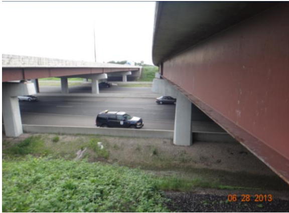
Figure 3.4.44: Bridge #19824 with roadway
