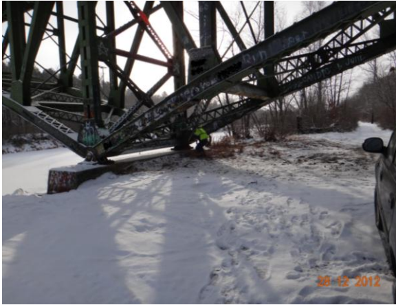
Figure 3.1.1: Bridge #5718 with waterway
