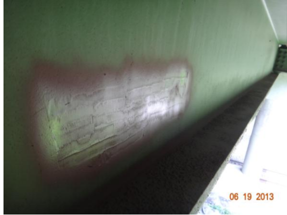
Figure 3.4.58: Bridge #27513 sampling location with roadway
