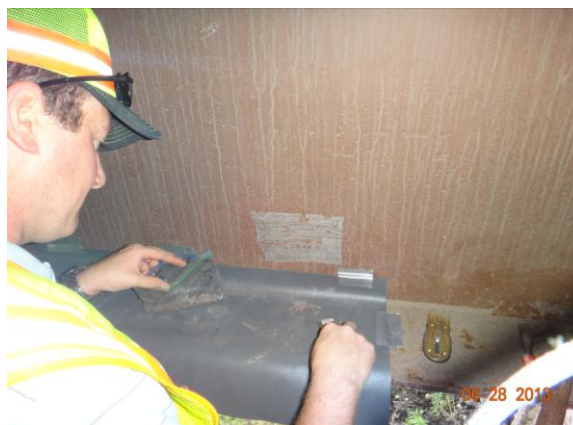
Figure 3.4.43: Bridge #19823 sampling location
