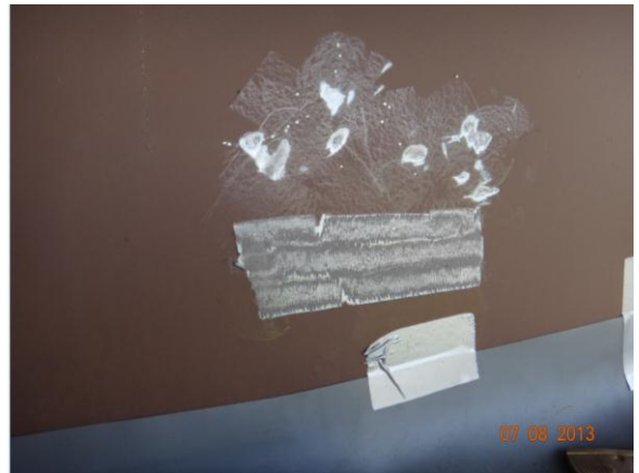
Figure 3.4.39: Bridge #9012 sampling location
