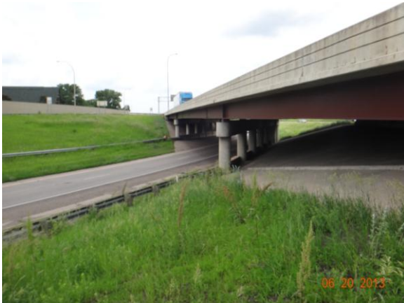
Figure 3.4.19: Bridge #27734 with roadway
