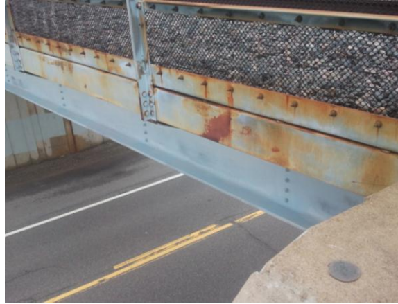
Figure 3.1.13: Bridge #9186 with roadway
