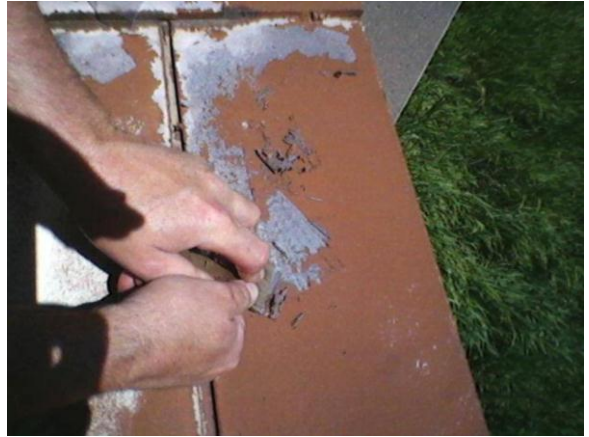
Figure 3.4.37: Bridge #9390 sampling location
