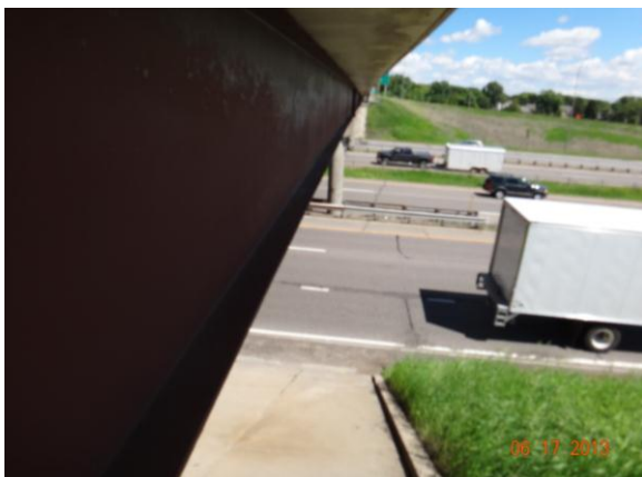
Figure 3.4.61: Bridge #27080 with roadway
