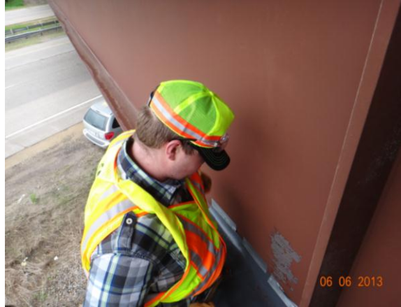
Figure 3.4.26: Bridge #82848 sampling location with roadway
