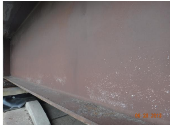
Figure 3.4.31: Bridge #82832 sampling location
