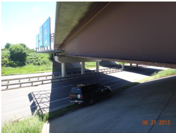
Figure 3.4.49: Bridge #19037 with roadway
