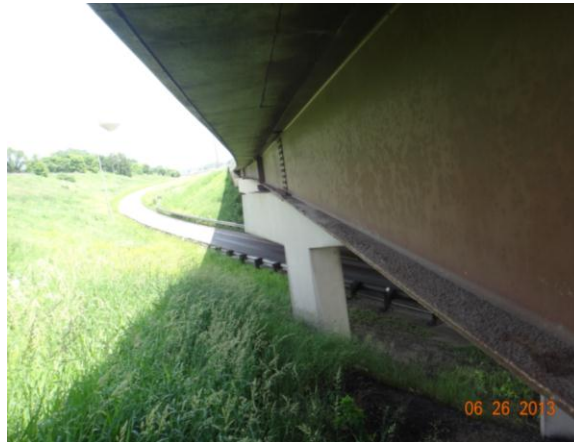
Figure 3.4.57: Bridge #19884 sampling location with roadway
