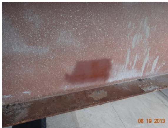
Figure 3.4.64: Bridge #27014 sampling location
