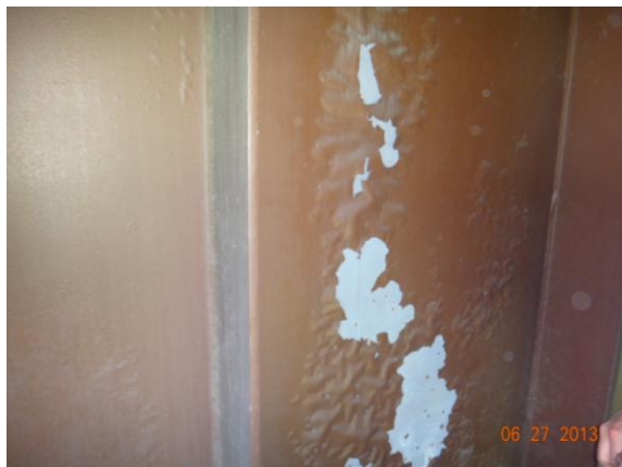
Figure 3.4.52: Bridge #19832 sampling location
