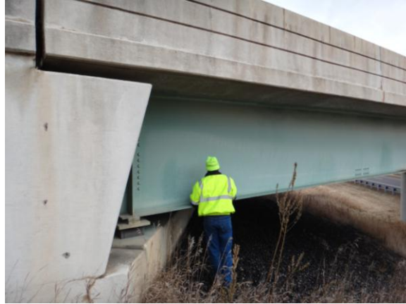
Figure 3.1.4: Bridge #9838 sampling location with roadway
