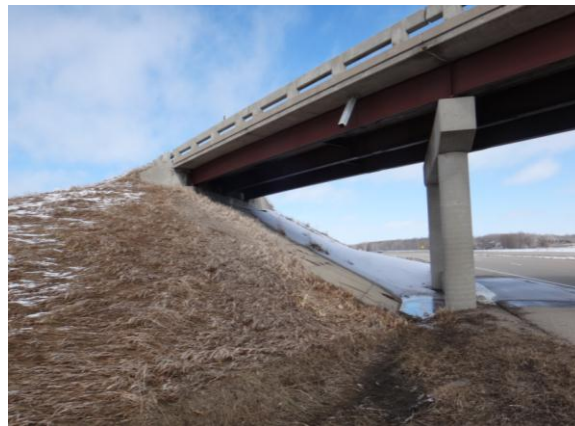
Figure 3.2.3: Bridge #73818 with roadway
