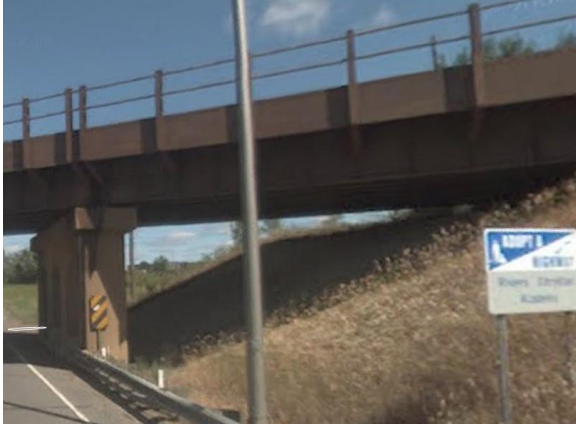
Figure 3.2.1: Bridge #9480 with roadway
