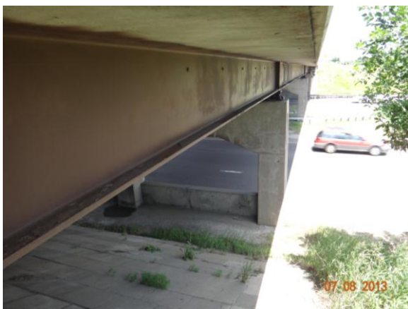
Figure 3.4.40: Bridge #9013 with roadway
