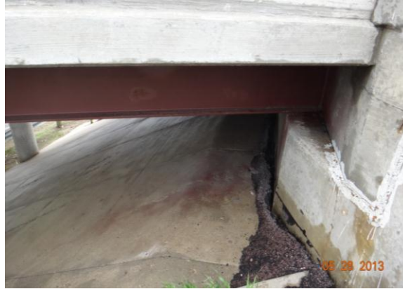
Figure 3.3.4: Bridge #67801 sampling location with roadway shoulder
