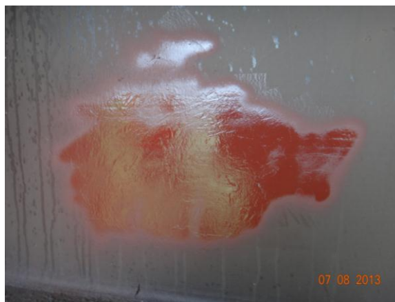
Figure 3.4.41: Bridge #9013 sampling location
