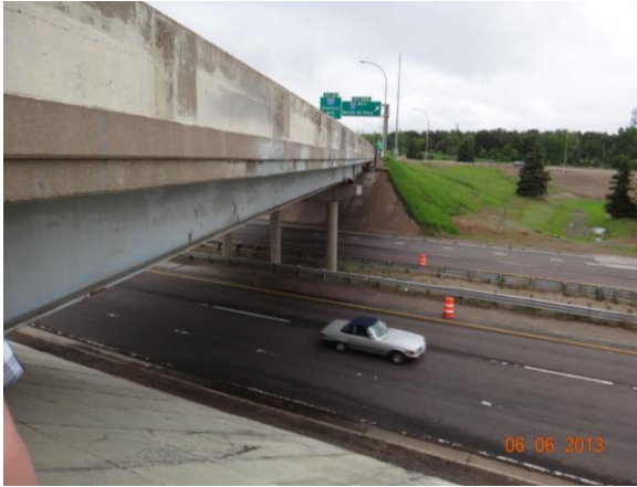
Figure 3.4.28: Bridge #82814 with roadway
