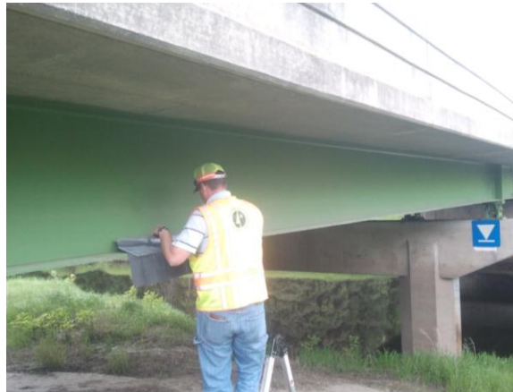
Figure 3.1.14: Bridge #6503 sampling location with waterway
