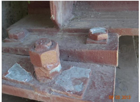
Figure 3.1.10: Bridge #69811 sampling location
