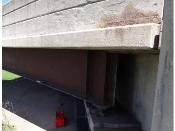
Figure 3.1.8: Bridge #69808A sampling location
