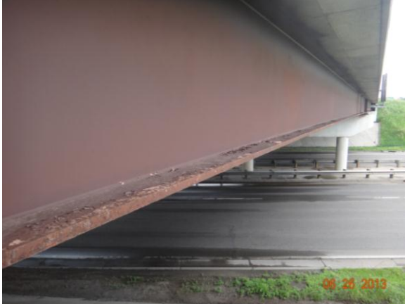
Figure 3.4.55: Bridge #19038 with roadway
