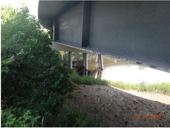
Figure 3.4.5: Bridge #27031A with roadway
