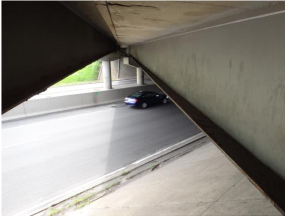
Figure 3.4.9: Bridge #27038 with roadway
