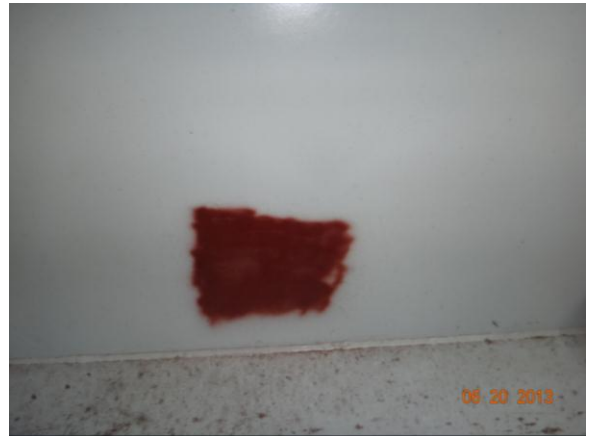
Figure 3.4.4: Bridge #27549A sampling location
