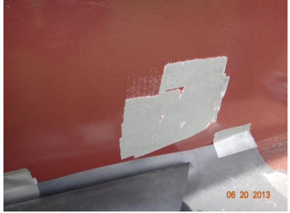
Figure 3.4.18: Bridge #27913 sampling location
