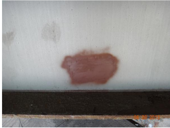
Figure 3.4.10: Bridge #27038 sampling location
