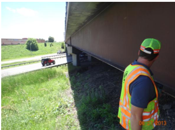
Figure 3.4.51: Bridge #19832 with roadway
