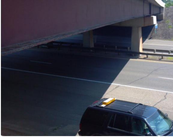
Figure 3.4.13: Bridge #82849 with roadway
