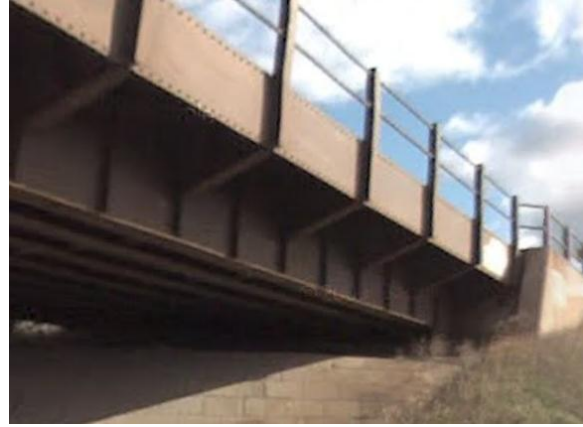
Figure 3.2.2: Bridge #9480 sample location
