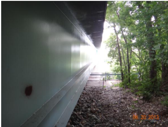
Figure 3.4.3: Bridge #27549A with waterway
