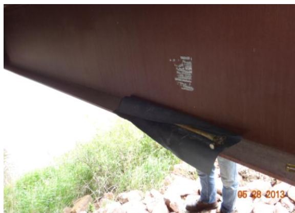
Figure 3.3.1: Bridge #67806 sampling location with waterway
