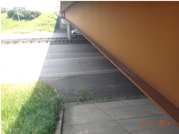
Figure 3.4.11: Bridge #27033 with roadway
