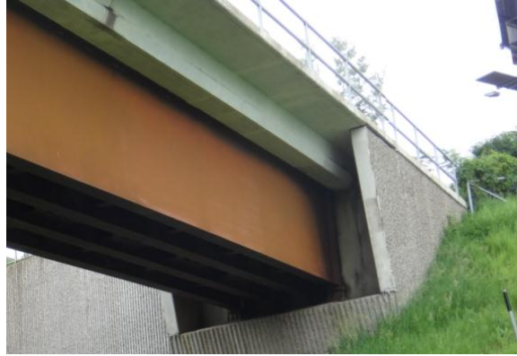
Figure 3.4.23: Bridge #19829 sampling location
