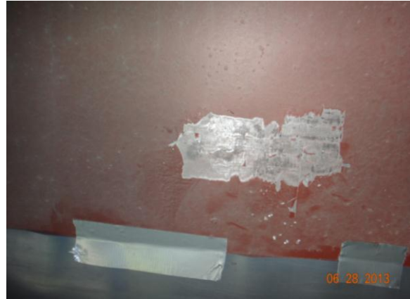
Figure 3.4.45: Bridge #19824 sampling location
