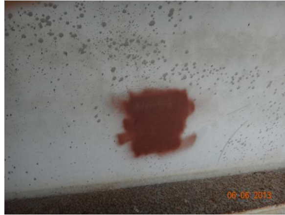
Figure 3.4.29: Bridge #82814 sampling location
