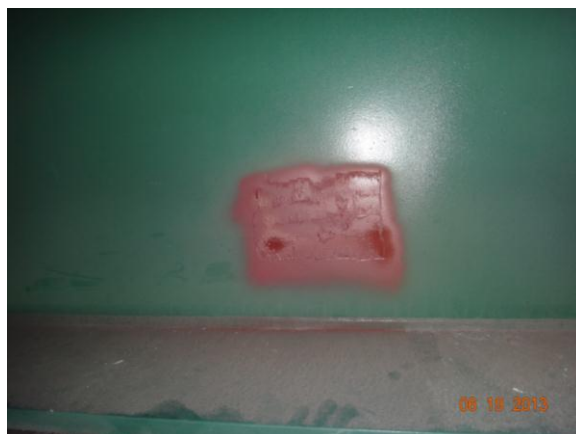
Figure 3.4.60: Bridge #27106 sampling location
