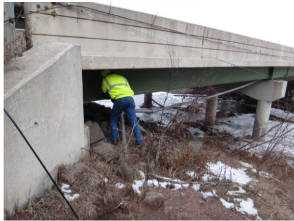
Figure 3.1.12: Bridge #9341 sampling location with waterway
