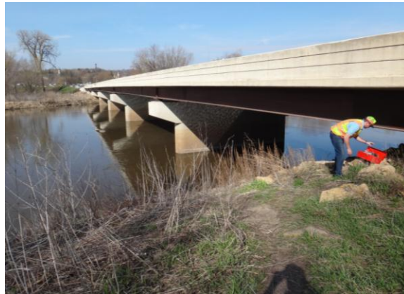
Figure 3.3.5: Bridge #40001 sampling location with waterway
