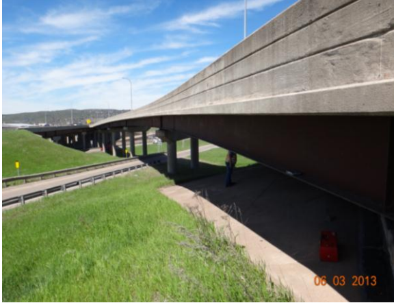
Figure 3.1.7: Bridge #69808A with roadway
