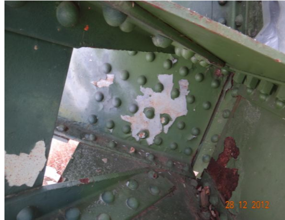
Figure 3.1.2: Bridge #5718 sampling location
