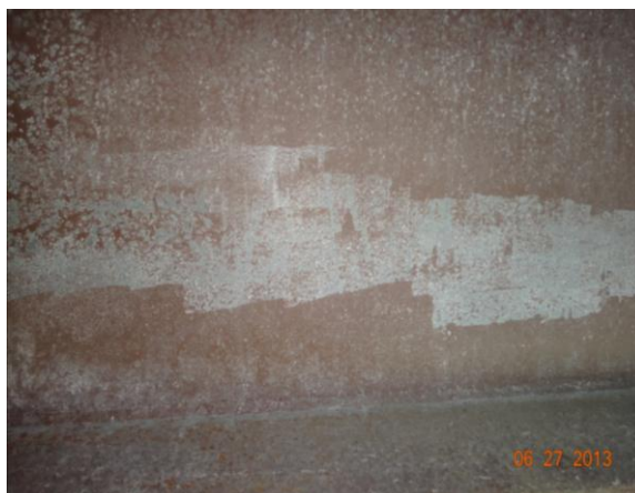
Figure 3.4.54: Bridge #19854 sampling location
