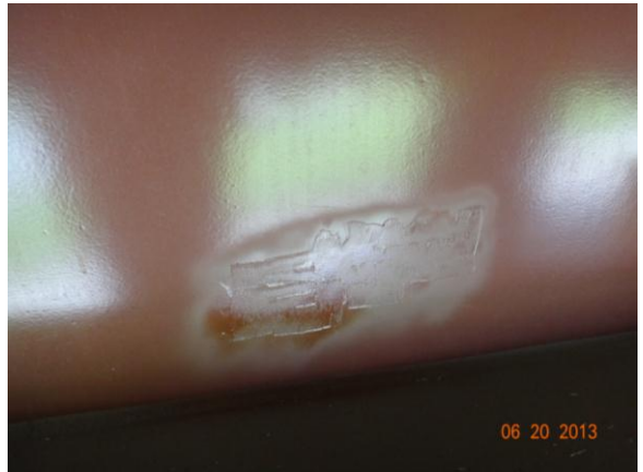
Figure 3.4.20: Bridge #27734 sampling location
