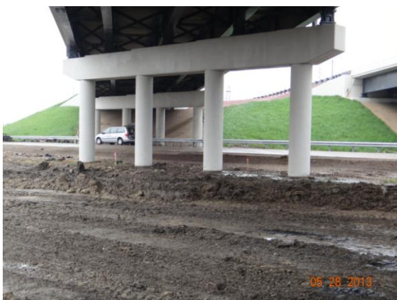
Figure 3.3.2: Bridge #53820 with roadway
