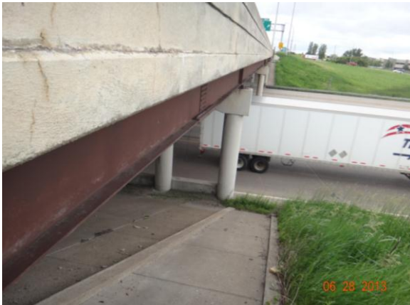
Figure 3.4.30: Bridge #82832 with roadway
