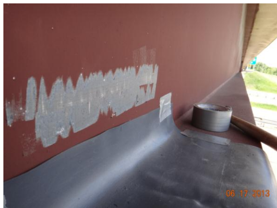
Figure 3.4.62: Bridge #27080 sampling location
