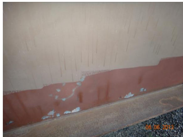
Figure 3.4.47: Bridge #19882 sampling location
