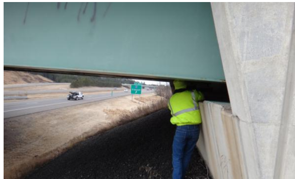
Figure 3.1.3: Bridge #9837 sampling location with roadway
