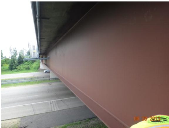
Figure 3.4.24: Bridge #82844 with roadway
