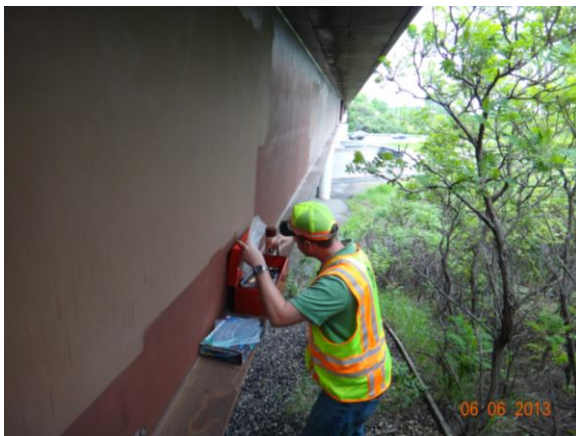
Figure 3.4.46: Bridge #19882 with roadway
