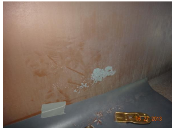
Figure 3.4.50: Bridge #19037 sampling location
