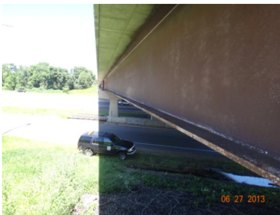
Figure 3.4.53: Bridge #19854 with roadway
