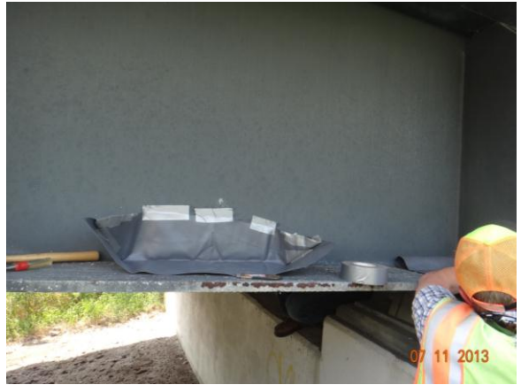
Figure 3.4.6: Bridge #27031A sampling location
