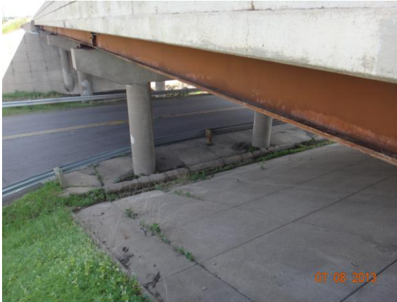
Figure 3.4.32: Bridge #9351 with roadway
