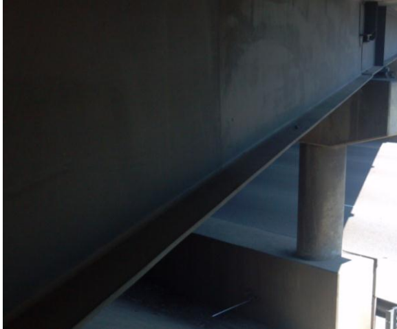
Figure 3.4.1: Bridge #27869 with roadway
