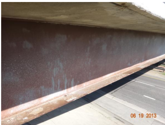
Figure 3.4.63: Bridge #27014 with roadway
