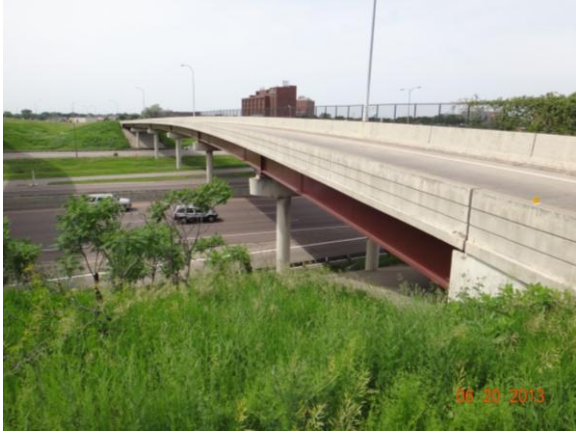
Figure 3.4.17: Bridge #27913 with roadway
