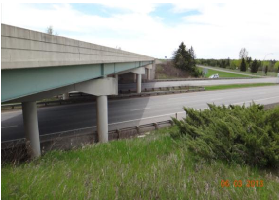
Figure 3.1.5: Bridge #9188 with roadway
