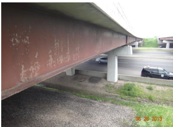
Figure 3.4.42: Bridge #19823 with roadway
