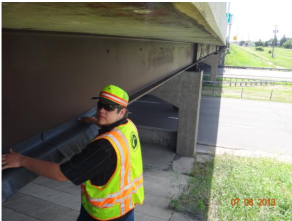
Figure 3.4.38: Bridge #9012 with roadway
