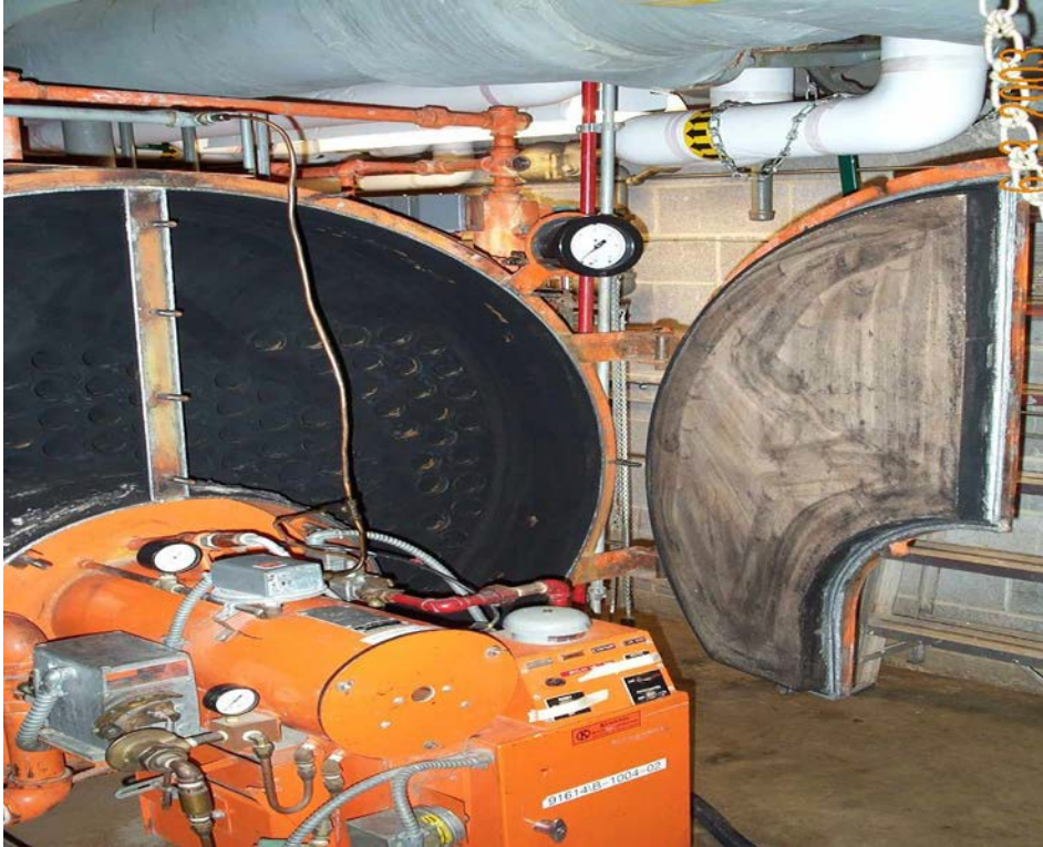
Boiler room with gray, crescent-shaped refractory mold visible against back wall.
