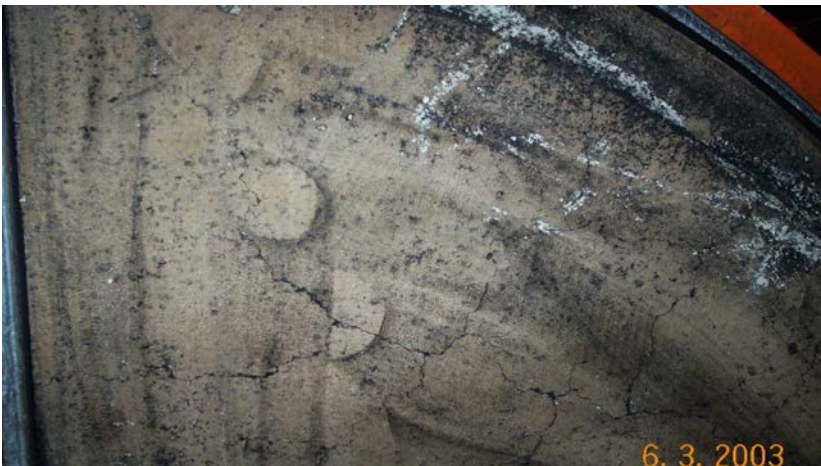
Boiler mold is cracking and in need of repair.
