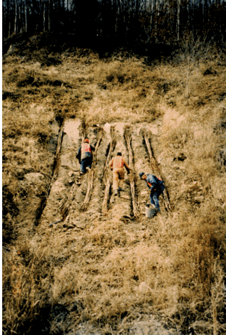
Placing wattles in the vertical drain trenches
