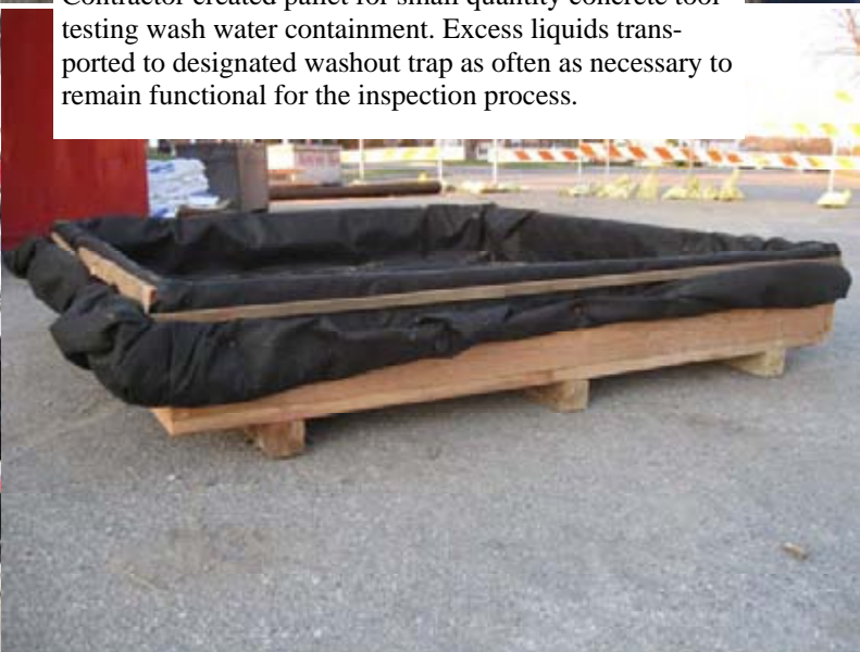
Concrete bucket washout and solids management placed in contractor developed containment box, maintained each day of ready mix operations.
