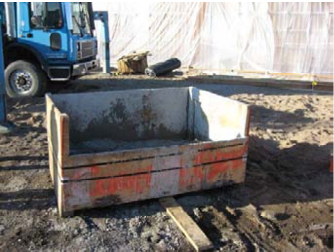
Sealed or plastic lined wood washout box
