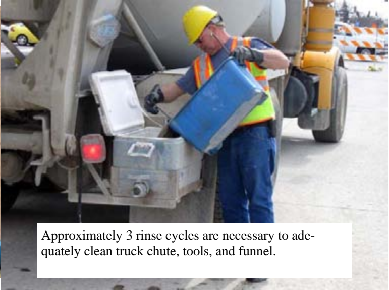
Plastic wash trough mounted with rebar hooks to chute, capable of containing rinse wash water and
