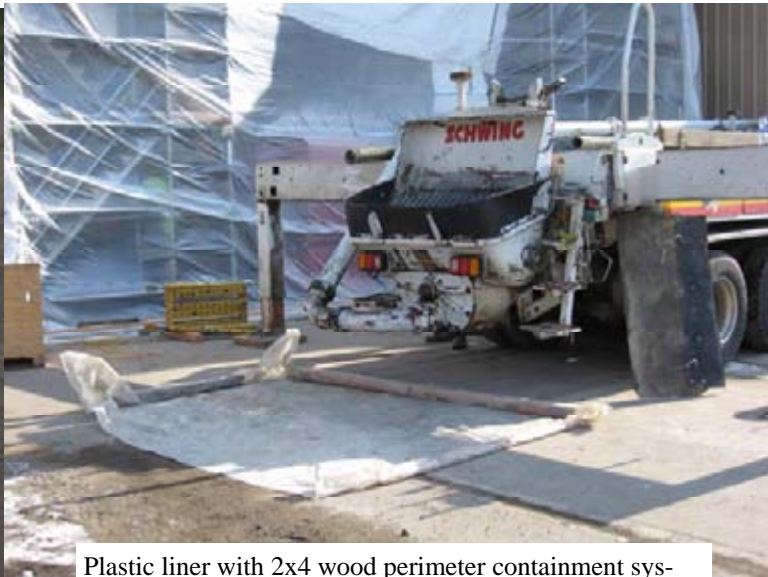
Plastic liner with 2x4 wood perimeter containment system during concrete transfer operations to pumper truck.
