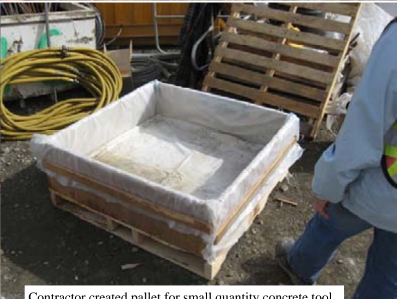
Contractor created pallet for small quantity concrete tool testing wash water containment. Excess liquids transported to designated washout trap as often as necessary to remain functional for the inspection process.
