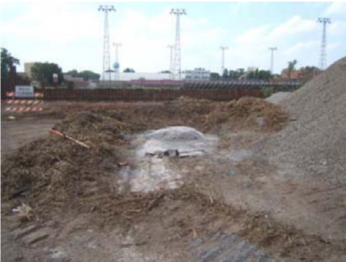
Slash mulch filter ring on low infiltration soils
