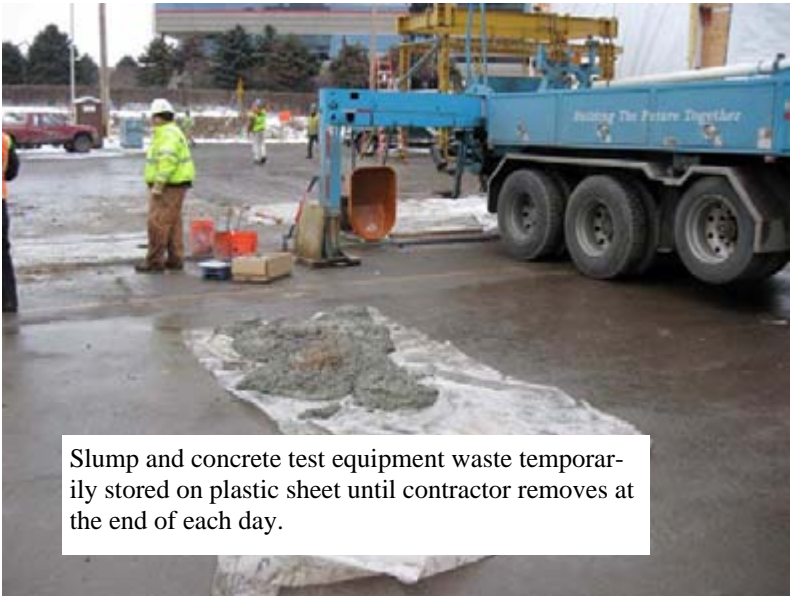
Small quantity concrete wash water into bermed plastic lined trap
