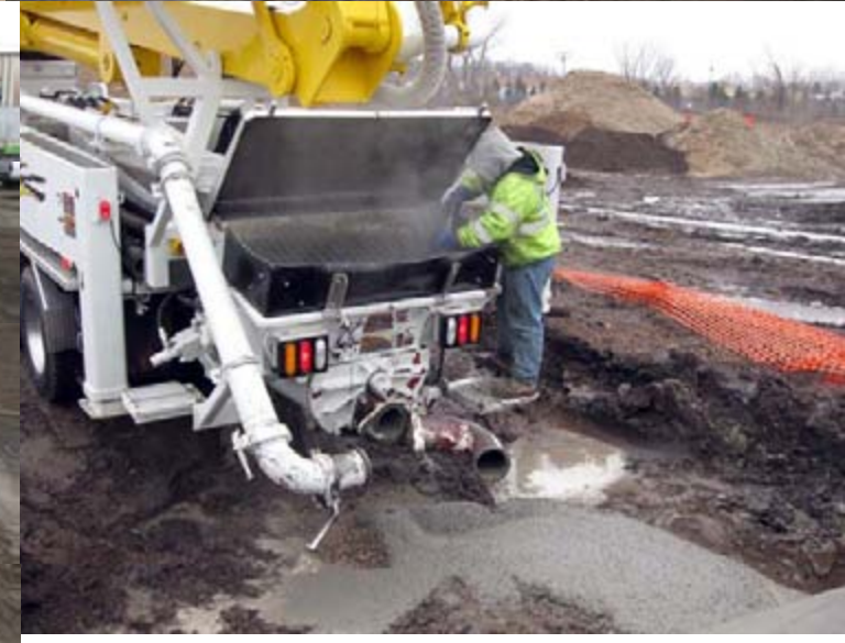
Final remnant of pumper hopper washout into designated and signed washout trap.
