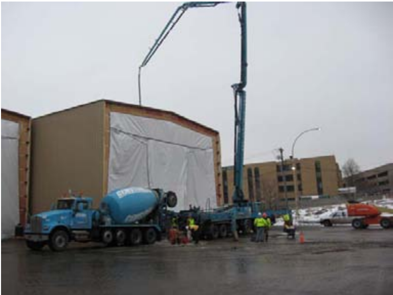
Pumper grout slurry discharge form box
