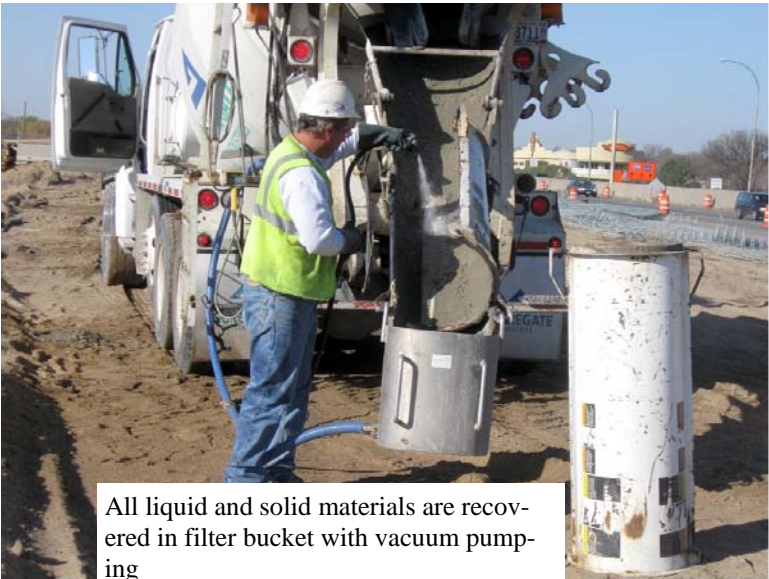
Chute funnel installed onto chute section, prior to lowering chute funnel port to tank opening.
