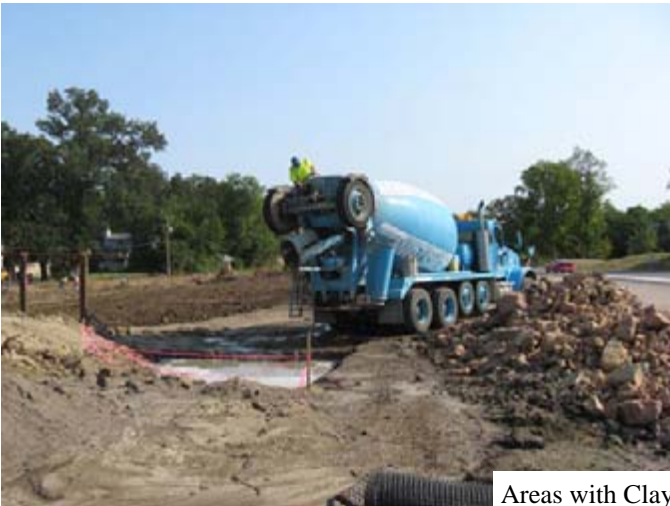
Areas with Clay soil that allow storage until evaporation of liquids
