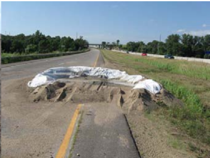
Mixing sand berm with plastic liner
