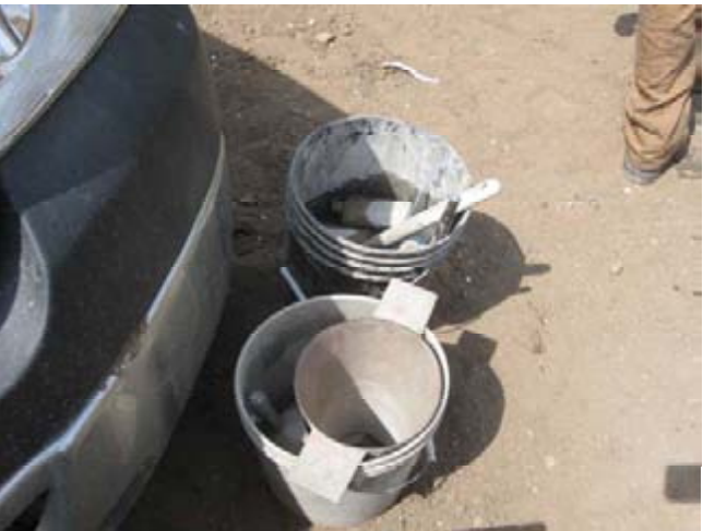
Small amounts less than 0.5 gallons may be disposed of on the grade if all material remains in the profile or evaporates prior to the next anticipated storm event. Sand may be used to absorb liquid wastes for later transport to the designated wash-out area.
