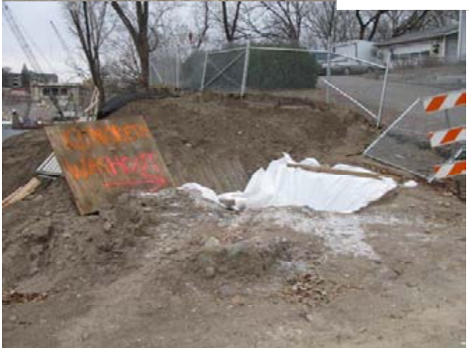
Plastic Liner with posted sign or spray painted notice for washout.
