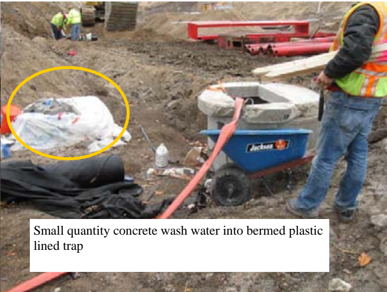
Traditional designated washout areas can be used for rinse water until evaporation.
