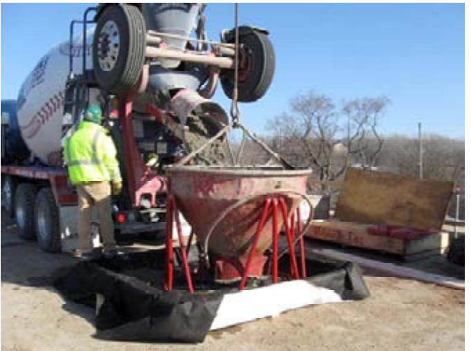
2x10 plastic and geotextile box, with 2x4 cleats for front loader pickup and movement
