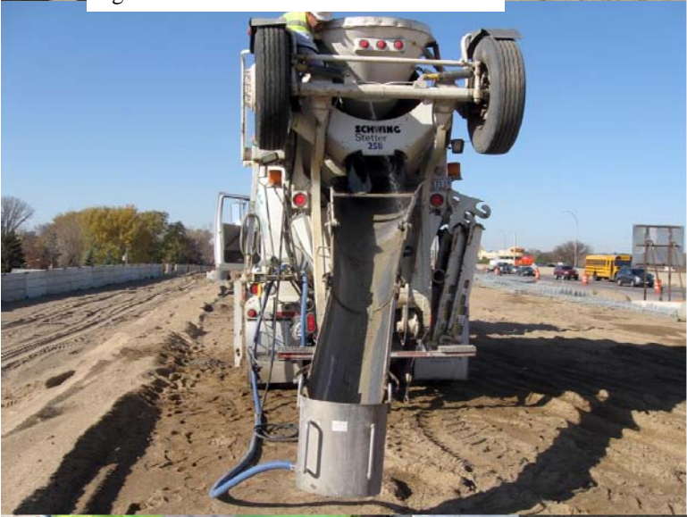
All liquid and solid materials are recovered in filter bucket with vacuum pumping
