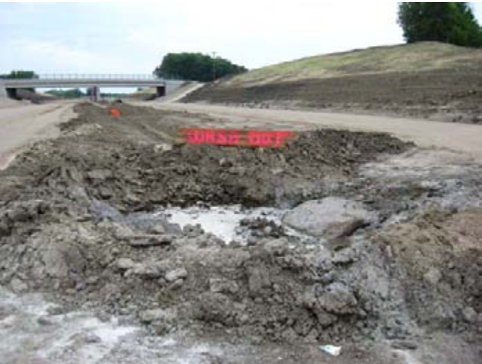
High cohesive, low infiltration soil berm
