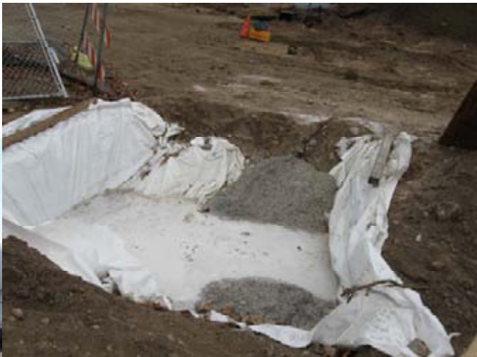
Plastic Liner with posted sign or spray painted notice for washout.
