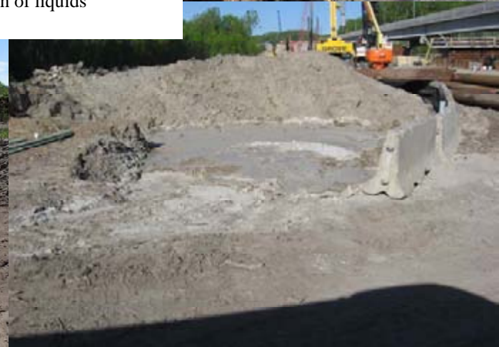
Areas with Clay soil that allow storage until evaporation of liquids
