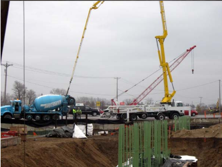
Priming or washing out of pumper truck into empty concrete truck for total containment of washout slurry.
