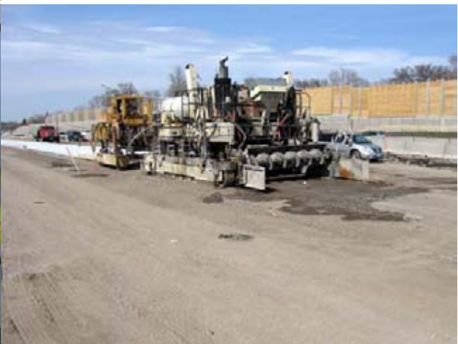
Small quantity wash water placed on grade where equipment washoff has been designated in the SWPPP, in areas to receive permanent pavements.
