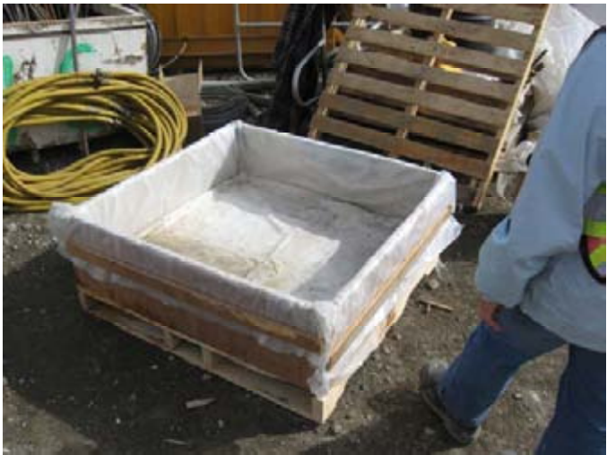
Sealed or plastic lined wood washout box
