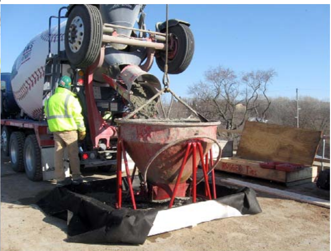
Concrete bucket washout and solids management placed in contractor developed containment box, maintained each day of ready mix operations.
