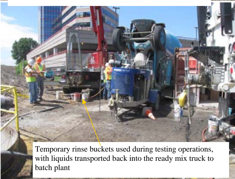
Small amounts less than 0.5 gallons may be disposed of on the grade if all material remains in the profile or evaporates prior to the next anticipated storm event. Sand may be used to absorb liquid wastes for later transport to the designated wash-out area.
