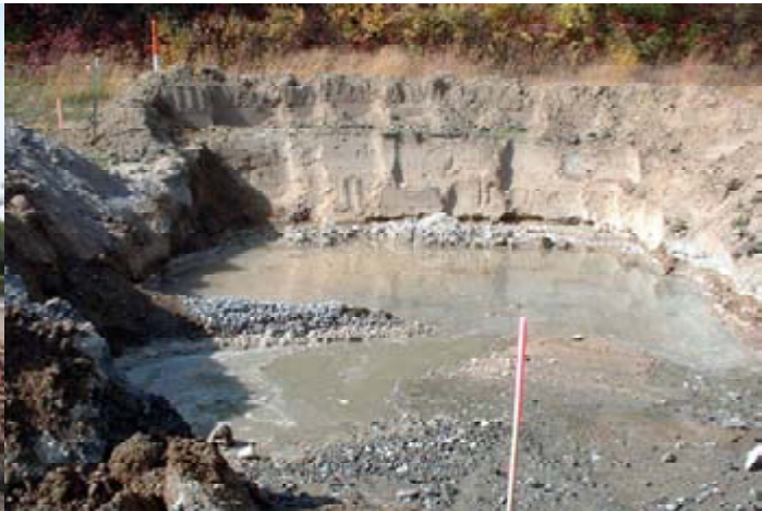
Areas with Clay soil that allow storage until evaporation of liquids
