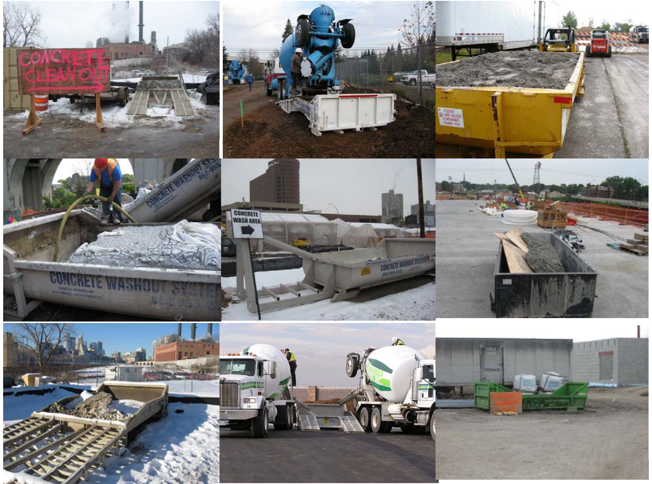
Various concrete liquid and solid dumpster systems sized to store all materials until liquid evaporates or vacuum removed and treated by commercial operators.
