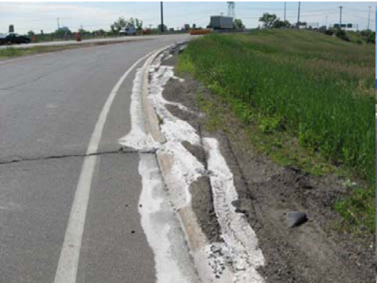
Washoff slurry must remain in gutter flow path by use of sand bags, rock logs or other best management practice above curb
