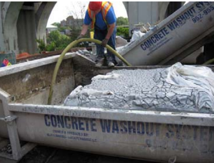
Sump trap must be cleaned as necessary by vacuum pump system, or managed by commercial concrete washout companies capable of handling slurry waste, treatment and transport.
