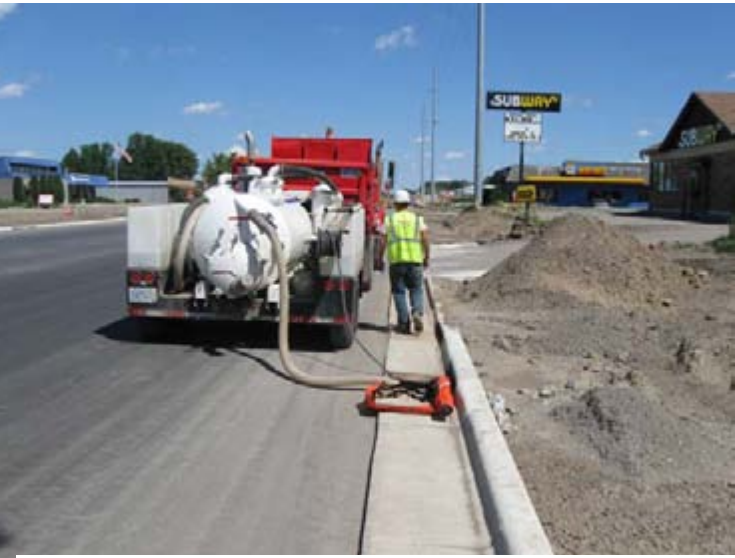
Sump trap must be cleaned as necessary by vacuum pump system, or managed by commercial concrete washout companies capable of handling slurry waste, treatment and transport.
