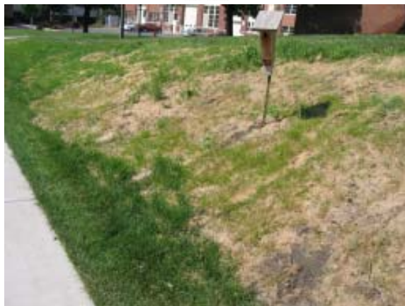
A blanket that has rapid degradable netting and stitching should be used in areas where mowing will take place
