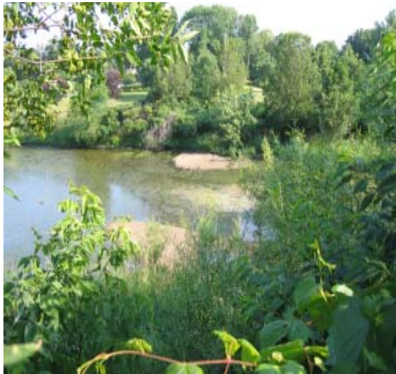
Stormwater pond with excess sediment
