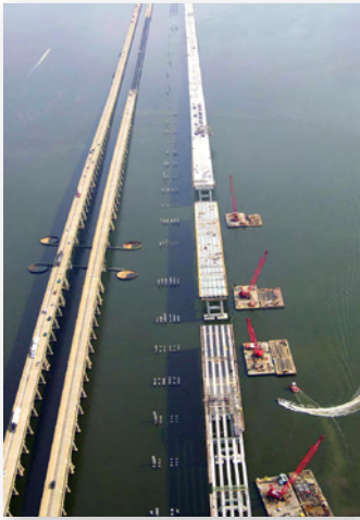
I-10 Bridges Pensacola - FLATIRON
