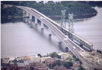
Sagadahoc Bridge - FLATIRON/FIGG
