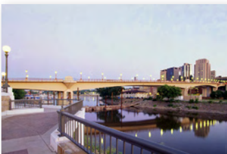
Wabasha Freedom Bridge -FIGG/TKDA
