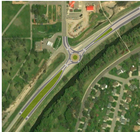
Roundabout at Chandler Ave
