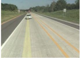
Figure 30 - Four-foot buffer with rumble strips
