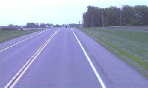
Figure 4 - Shoulder (edgeline) and centerline rumble strips
