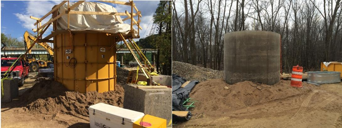
Technique Shaft SCC trial pour. Exterior forming system (left) and finished concrete (right).
