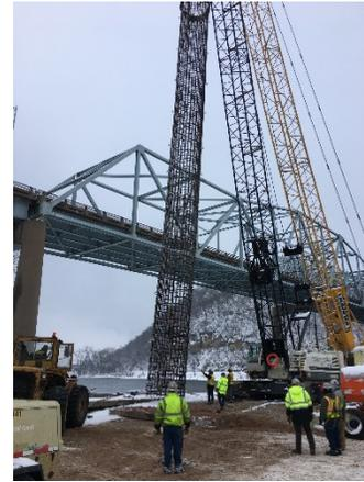
Technique Shaft Construction with casing cleanout (left) and rebar cage installation (right).
