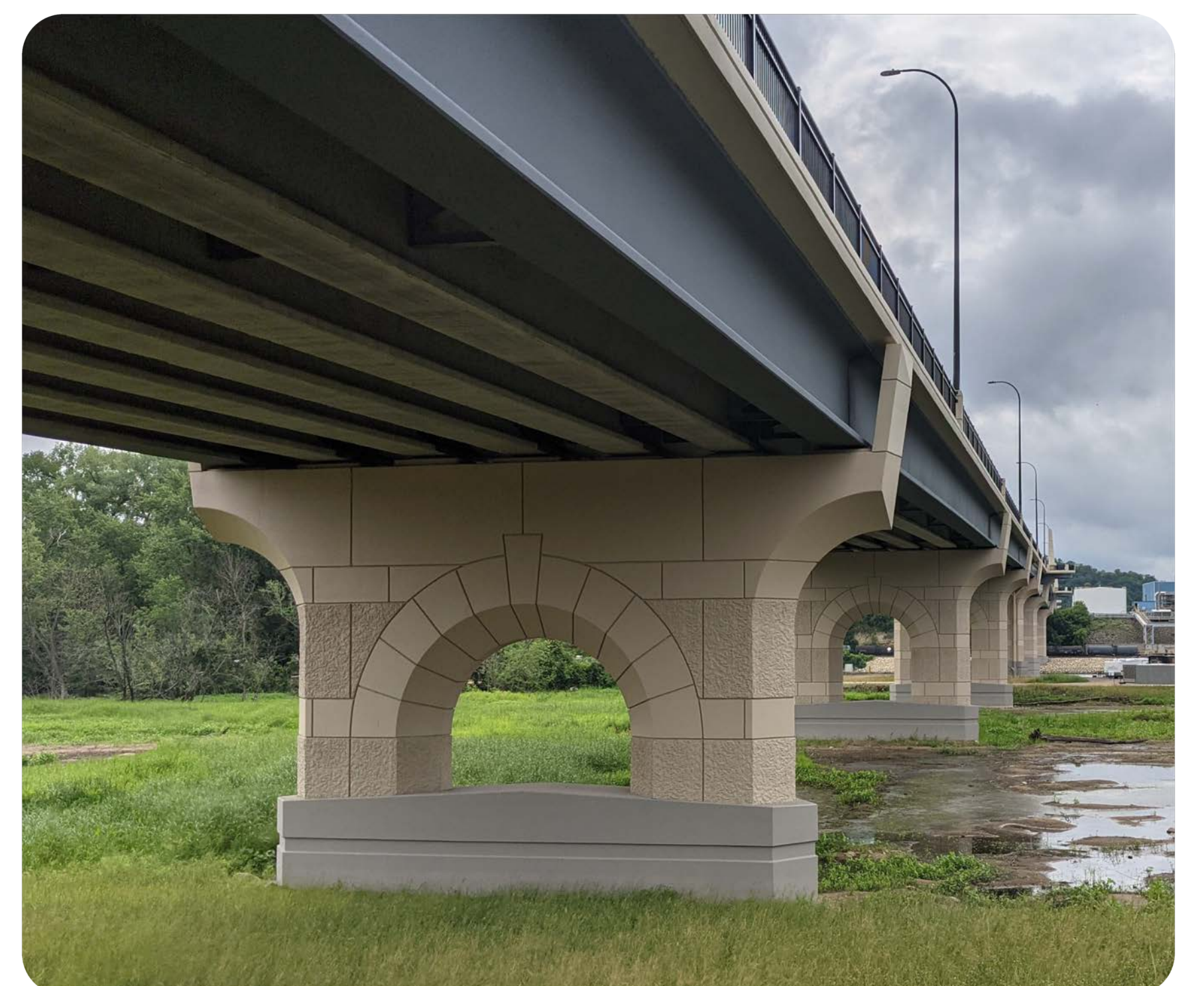
New Hwy 63 over the Mississippi River Pier Design
