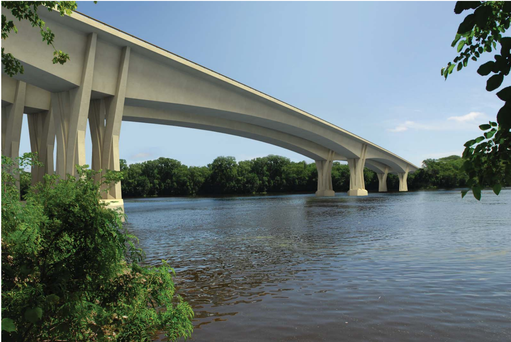
Proposed River Bridge Main Span and Piers Viewed from the Minnesota Bank
