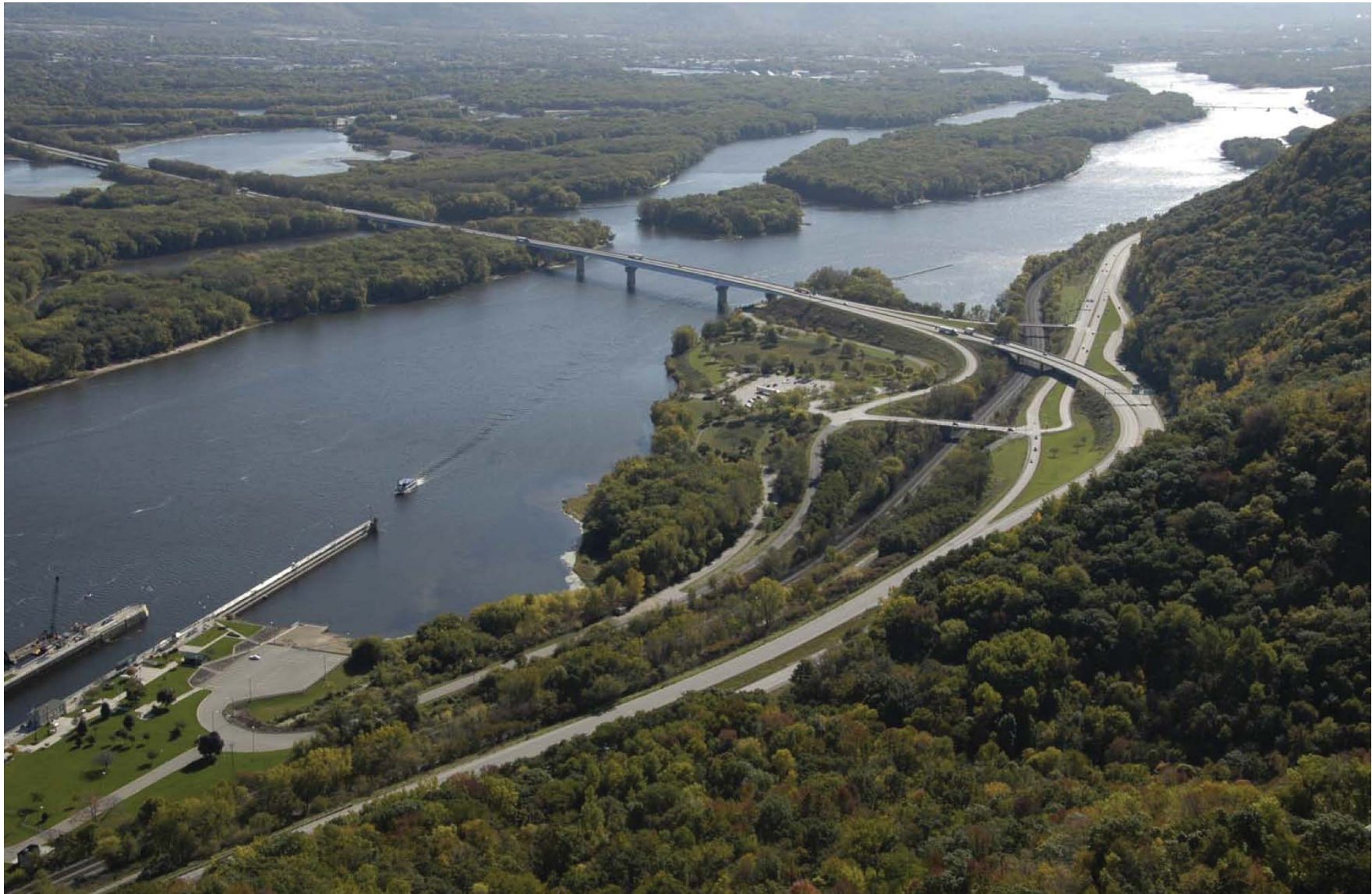
Aerial View of the Existing Minnesota Interchange
