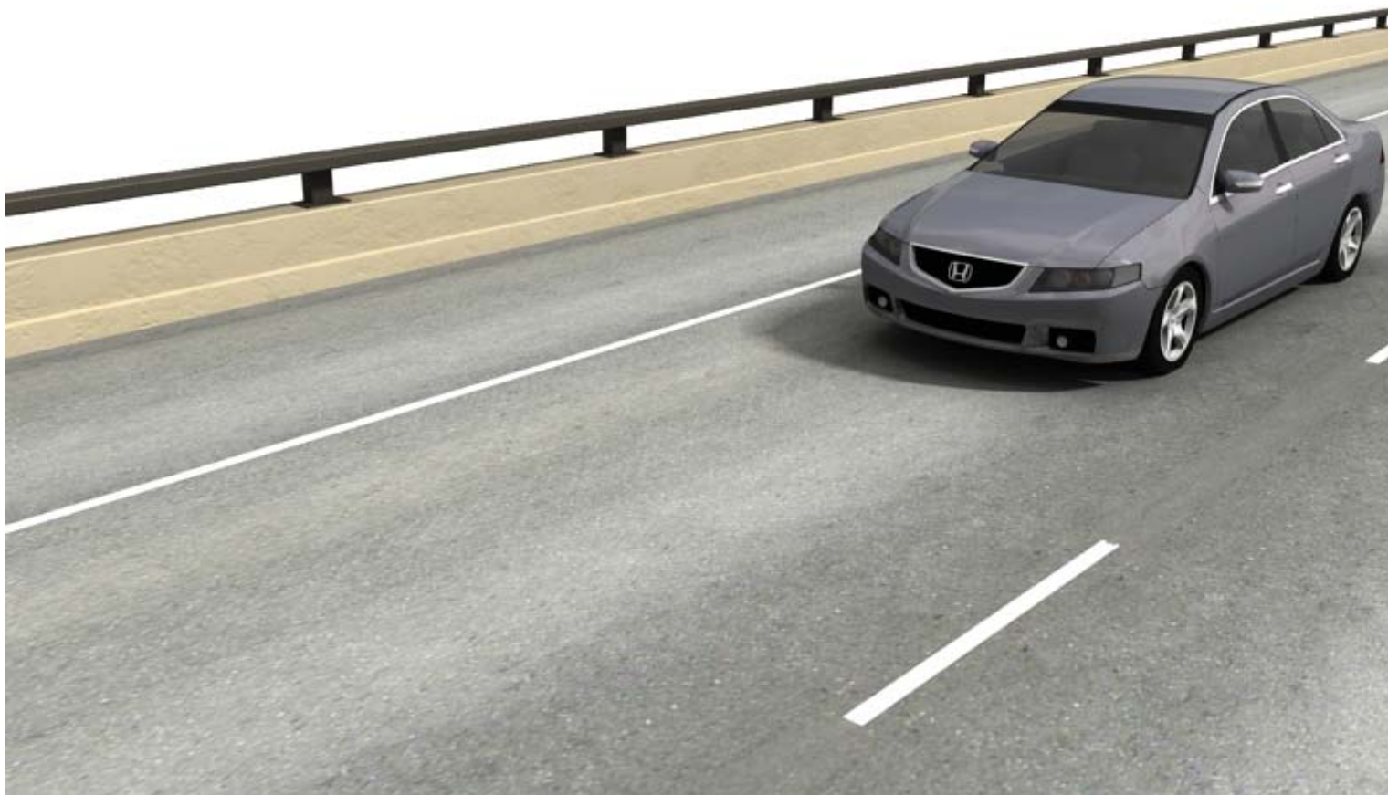
Open Tube Rail on River Bridge Allows for Views of the Surroundings
