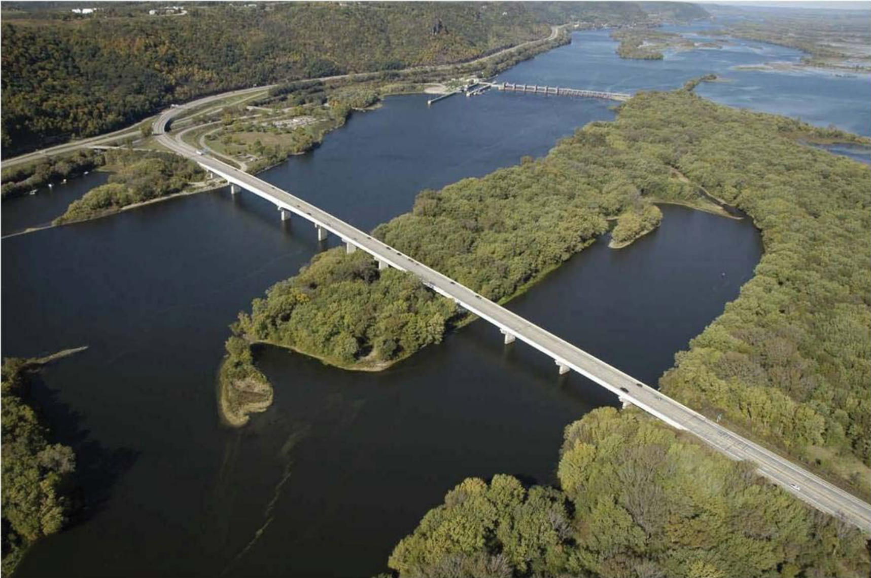
Aerial View of the Existing River Bridge and Approaches
