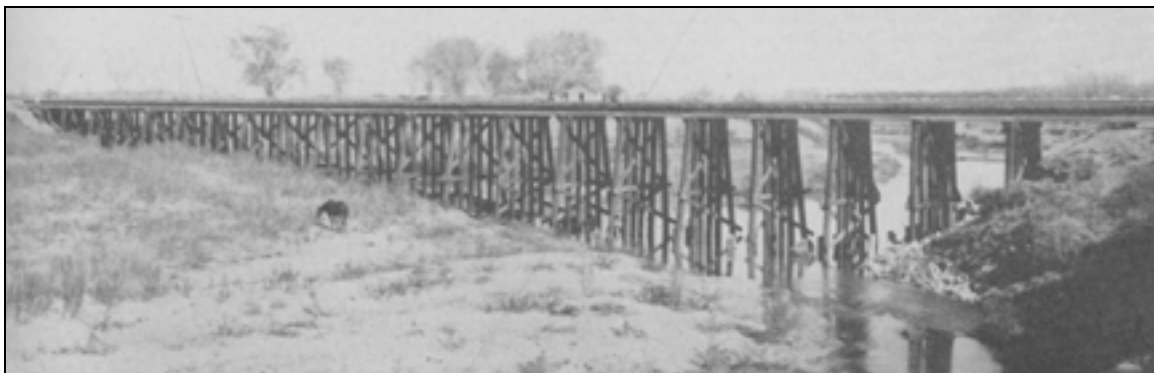
Figure 14. Typical pile trestle bridge (Howson 1926:527)
