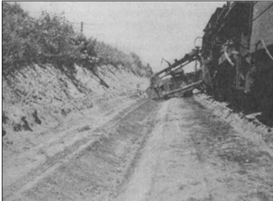
Figure 11. Construction of drainage ditches (Rench 1946:21)
