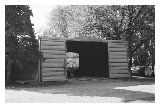
For much of the year this building is used as a granary, and after the grain is sold it stores vehicles and equipment until the next harvest. The steel's deep corrugation makes the structure strong and self-supporting. The building likely came in prefabricated sections that were bolted together. Retzlaff Farm, Framnas Township, Stevens County, 2004. (Gemini Research photo)
