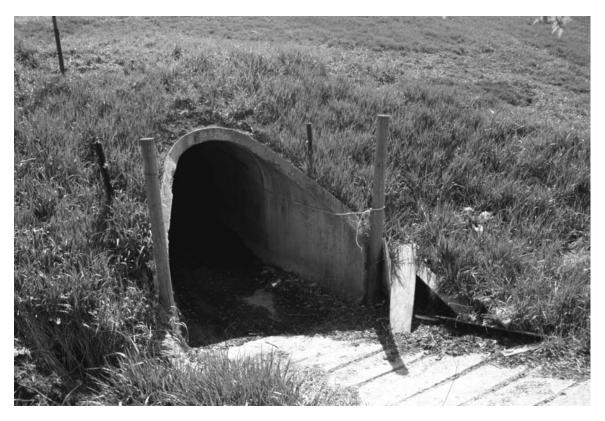
This poured concrete animal underpass in central Minnesota is approached by a scored concrete walkway. The walkway provides traction for animals and reduces erosion on the steep slope. Stearns County, 2004. (Gemini Research photo)
