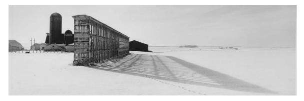
The optimal width for Minnesota corncribs was 6' to 7' but the length could vary. The height was determined first by comfortable hand-filling and then by the height of mechanical conveyors. This long, continuous crib probably had several interior partitions. Corncribs were often aligned north and south to catch cross-winds. Farm near LeCenter, 1998. (MHS photo by Chris Faust)
