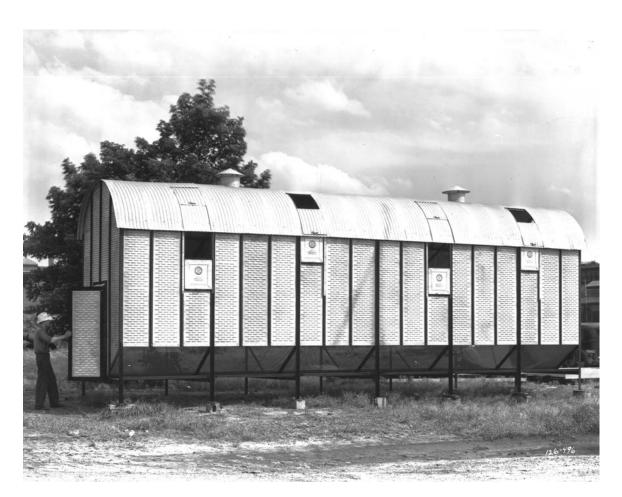
Prefabricated metal corncribs similar to this one were termed "experimental" in 1940 by *Successful Farming* magazine and the first models were just being marketed (Fox 1940). This version had perforated metal walls, which didn't ventilate as well as walls of wire mesh. Location unknown, photo 1938. (MHS photo by Norton and Peel)
