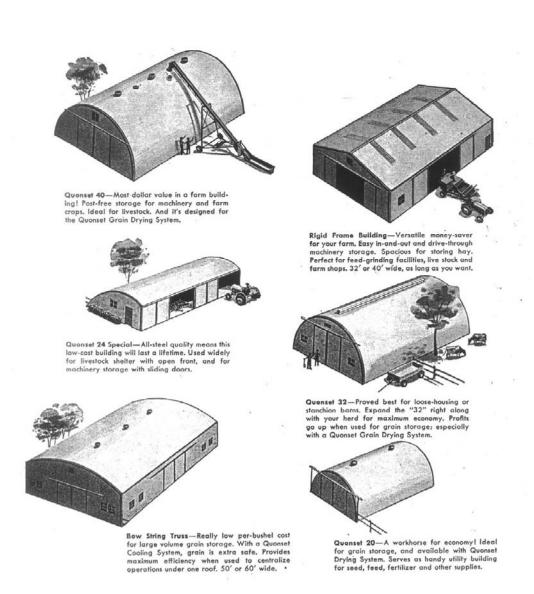
In 1957 Stran-Steel's line of buildings – including the "Quonset" brand – was marked for implement sheds, work shops, livestock barns, grain drying and storage, etc. Metal buildings tended to be cold and damp for livestock so were sometimes lined and insulated. The Stran-Steel Corporation had a regional office in Minneapolis. From *Agricultural Engineering* (Feb. 1957).
