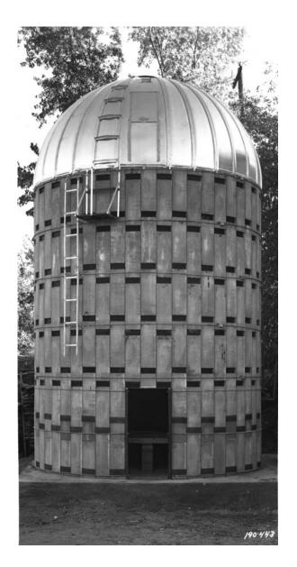
Cement stave corncribs were first built in the 1910s. This brand new example was photographed in 1949. It had steel reinforcing hoops, a hatch in the roof for filling, and a lower door for unloading – all typical of the type. The staves incorporated small metal grates that kept rodents from passing through the air gaps. Location unknown, 1949. (MHS photo by Norton and Peel)
