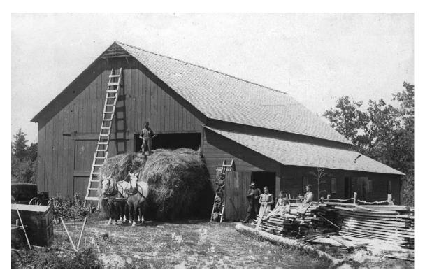
This barn in a cutover region is faced with vertical boards that were probably cut on or near the farm. (The shed-roof addition is faced with shiplap, likely purchased.) At right, the three girls are sitting on a large stack of thick, newly-cut boards. Morrison County, circa 1900. (MHS photo by Brooks)
