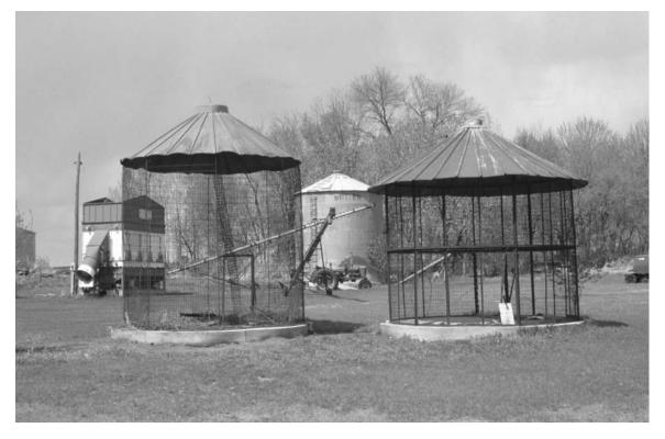
Two versions of prefabricated steel wire corncribs. Both have poured concrete floors and standing-seam metal roofs. Some cribs filled with ear corn can still be encountered in Minnesota. Stearns County, 2004. (Gemini Research photo)
