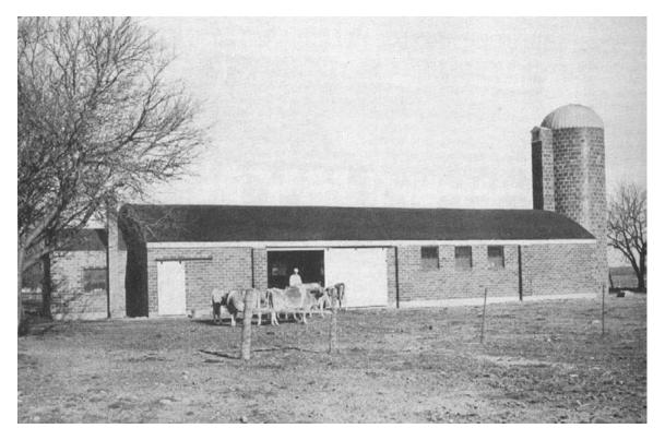
A one-story dairy barn and attached silo, both built of structural clay tile. Tile was usually glazed on one side to provide a sanitary, waterproof, cleanable interior for the barn, milk house, and silo. From *Dairy Cattle and Milk Production* by the University of Minnesota's Clarence H. Eckles (1950).
