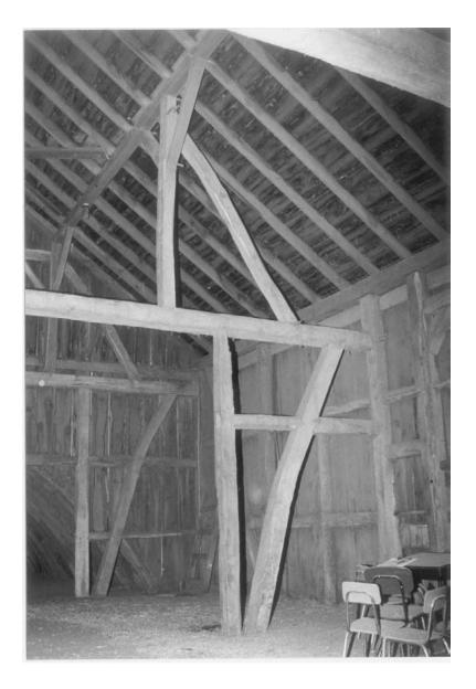
A circa 1880 timber frame barn built on a German immigrant farm in Nicollet County. The barn displays rare Old World construction techniques including plate-to-floor diagonal braces, use of curved timbers, scribed joinery, and fachwerk-style square framing of the exterior walls. Seeman Farm, Courtland Township, Nicollet County, 2005. (Photo by Daniel R. Pratt for Mn/DOT)
