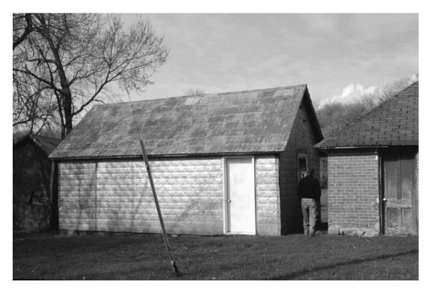
This farm building was sheathed in steel sheets stamped with a rockfaced masonry design – the most popular special pattern. The roof of the building was covered with a corrugated version. Iron and steel sheets were widely used to renew the appearance of woodframe and wood-sided buildings, and were sometimes the original exterior material. Grove Township, Stearns County, 2004. (Gemini Research photo)
