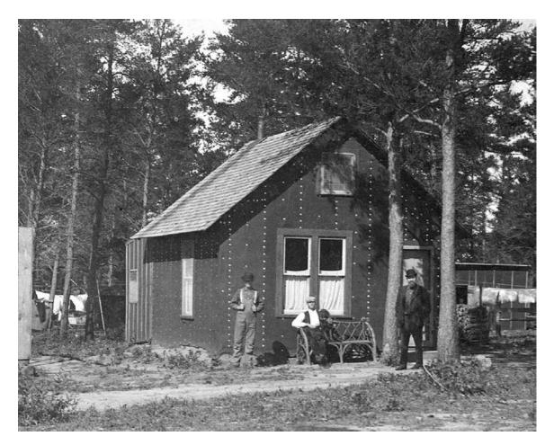
A farmhouse and outbuilding covered with tar paper, a common sheathing material that was inexpensive and readily available. The paper easily came loose with conventional nails, so it was secured with wide-headed tacks or strips of lath. It lasted longer in wooded areas where the trees offered some protection from the wind. Asphalt roofing material, available in shingles or rolls, was a more durable alternative. Cass County, circa 1910. (MHS photo)
