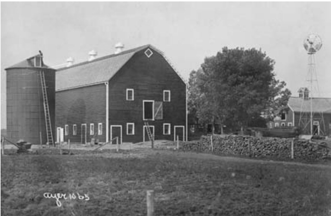
The wooden stave silo was being shingled when this photo was taken, and both the silo and the adjacent barn look new. Firewood and building materials are stacked in the farmyard. Hackney Farm, Ramsey County, circa 1910. (MHS photo by Harry Darius Ayer)
