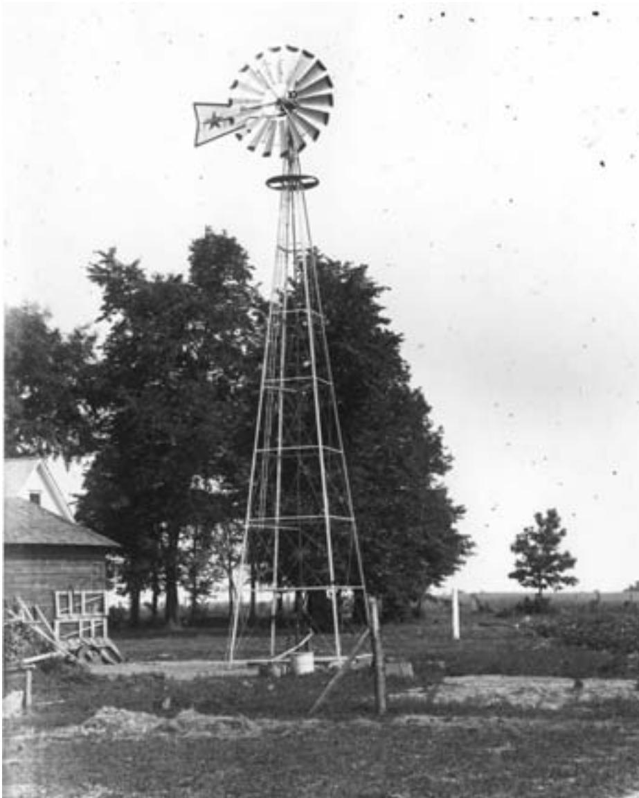
Steel windmills were introduced in the late 19th century and became common on Minnesota farms in the 1920s. This may be a Star windmill, identified by the star on the vane and the painted blade tips. The narrow ladder on the tower was used to service the gears and blades. Location unknown, circa 1910. (MHS photo)
