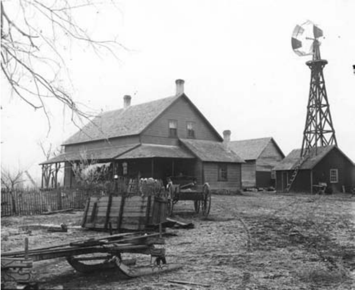
Sectional-wheel windmills had adjustable blades that folded inward as the wind speed increased, protecting the wheel and gears from damage. In early windmills, both blades and tower were built of wood. Some windmills were built on top of small buildings. Location unknown, circa 1900. (MHS photo by Joseph Jay Brechet)
