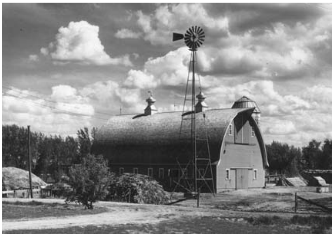
Solid-wheel windmills did not have folding blades, but were instead governed by a side vane that turned the wheel out of the wind when the velocity grew too great. Location unknown, circa 1930. (MHS photo)
