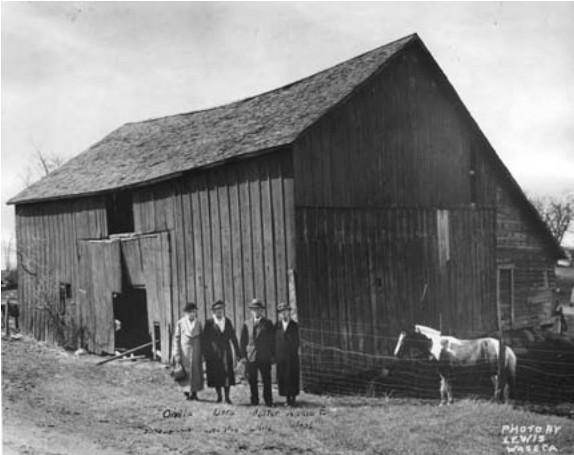
This threshing barn was apparently built in 1855 on the Childs Farm in Waseca County. After the farm diversified, the barn was altered to support animal husbandry. Wilton Township, Waseca County, 1938. (MHS photo by Lewis)
