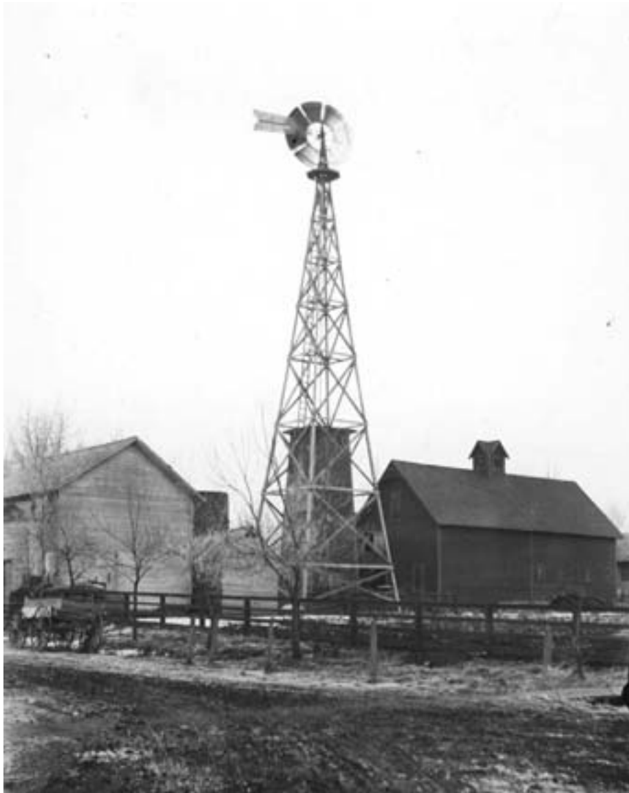
This farm windmill was fairly tall. (The height was in part determined by the height of trees on the farmstead.) A wooden silo is visible behind the windmill tower. Location unknown, circa 1900. (MHS photo by Joseph Jay Brechet)
