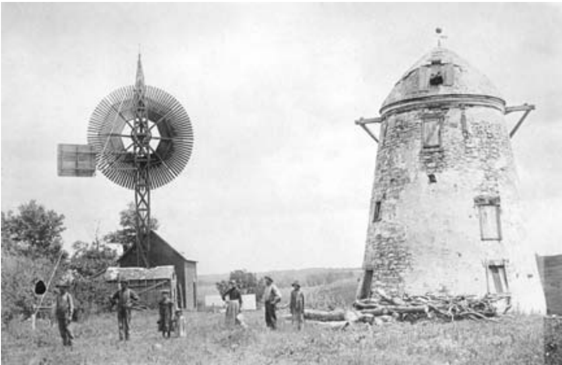
The towers of European-style windmills, like the Seppman Mill near Mankato (shown here), had to be sturdy enough to support the massive turning blades. They were used to grind grain. Circa 1890. (MHS photo)
