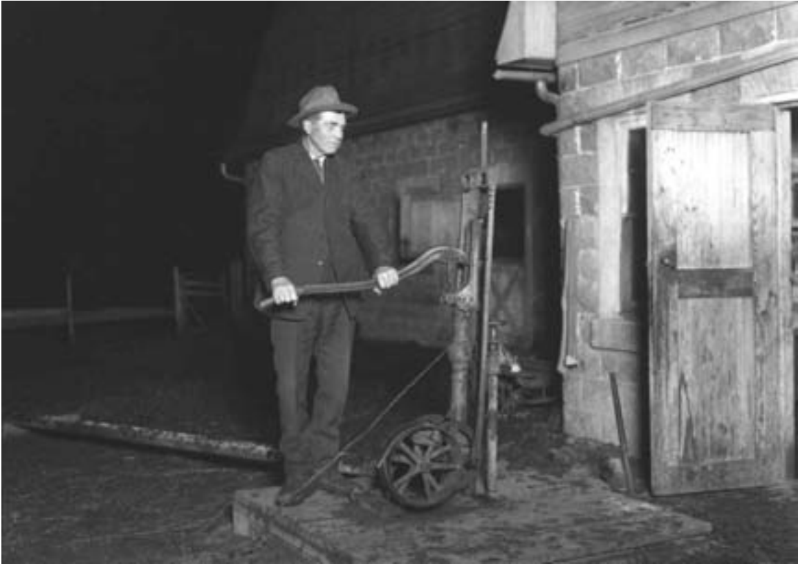
This well had a wooden cover and a hand pump, and was sited near the livestock. Kandiyohi County, circa 1920. (MHS photo)
