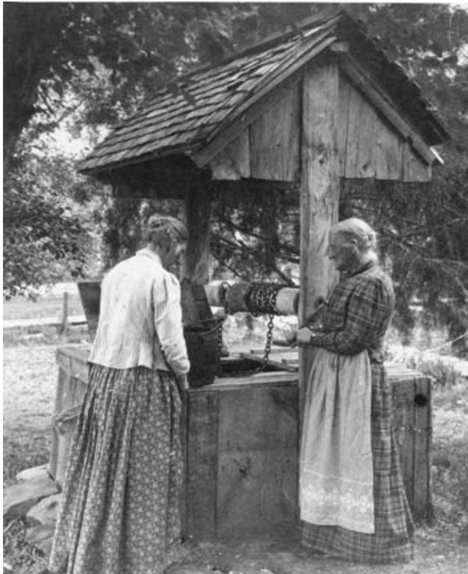
Using a windlass, rope, and bucket was a simple but labor-intensive way to raise water from an early farm well. Mechanical pumps soon became the preferred method. Photo taken near Marine-on-St. Croix, circa 1900. (MHS photo)
