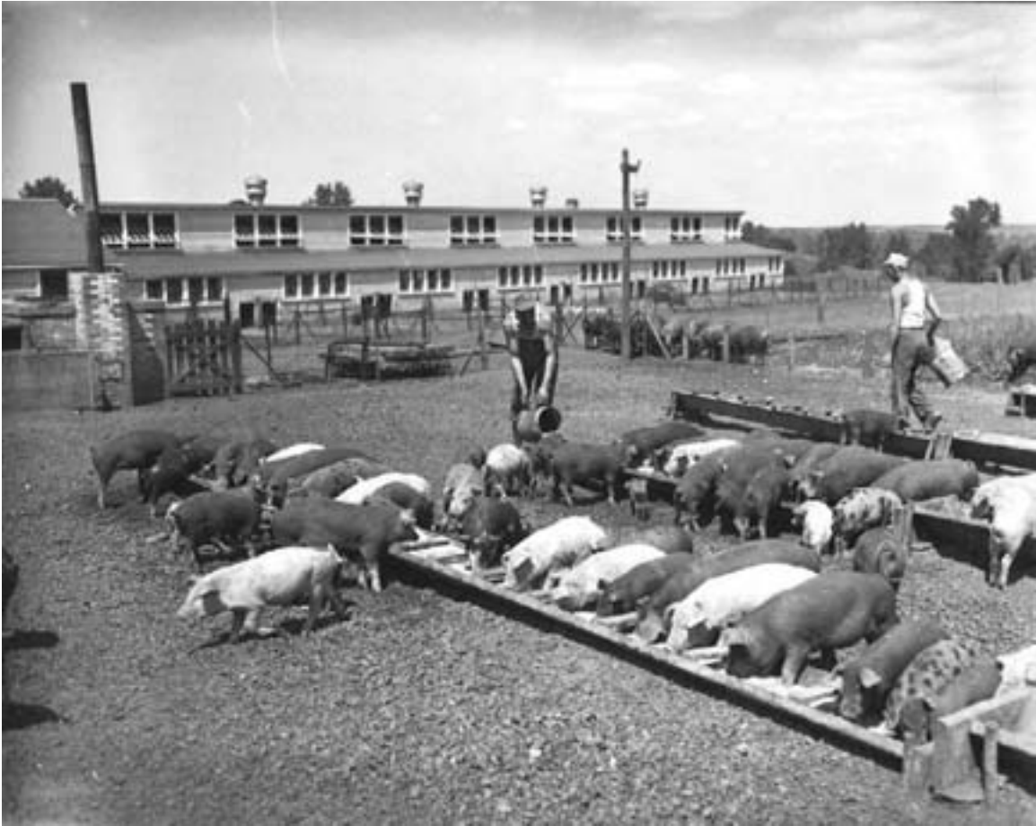
This pig barn had windows in the side walls and in the monitor to light two rows of stalls. The pigs ate at low, wooden troughs. The yard was surrounded by steel woven wire fencing (also called "hog wire" fencing). The brick structure with a stovepipe (at left edge) was probably a feed cooker. Farm possibly near Stillwater, 1940. (MHS photo by Minneapolis Star Journal )
